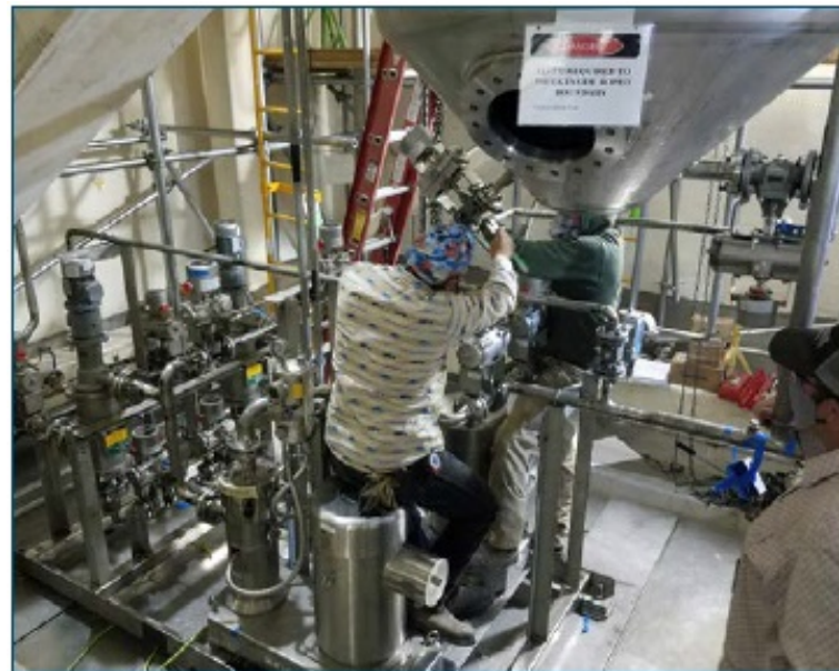
Torquing components on Wet Decon Skid
