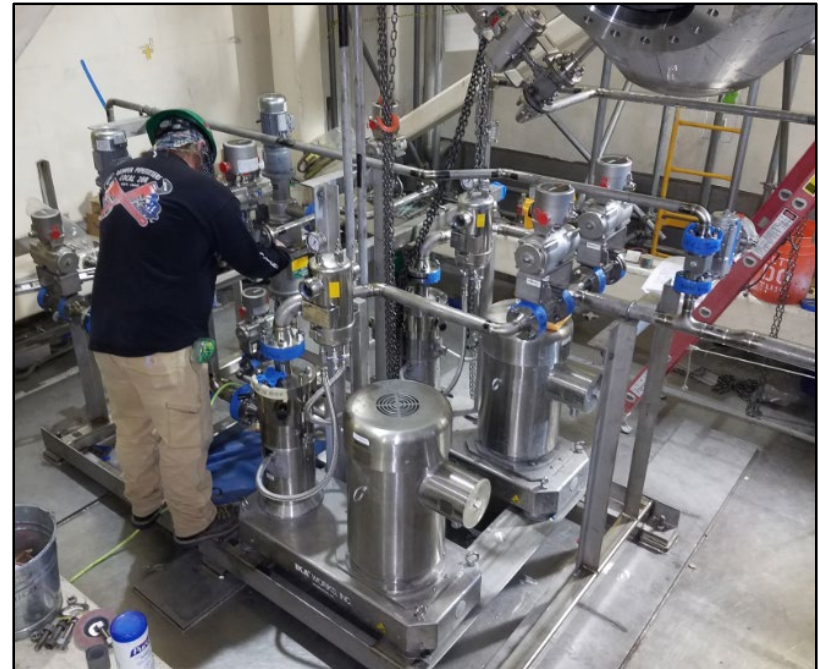
Wet Decon System Skid Installation
