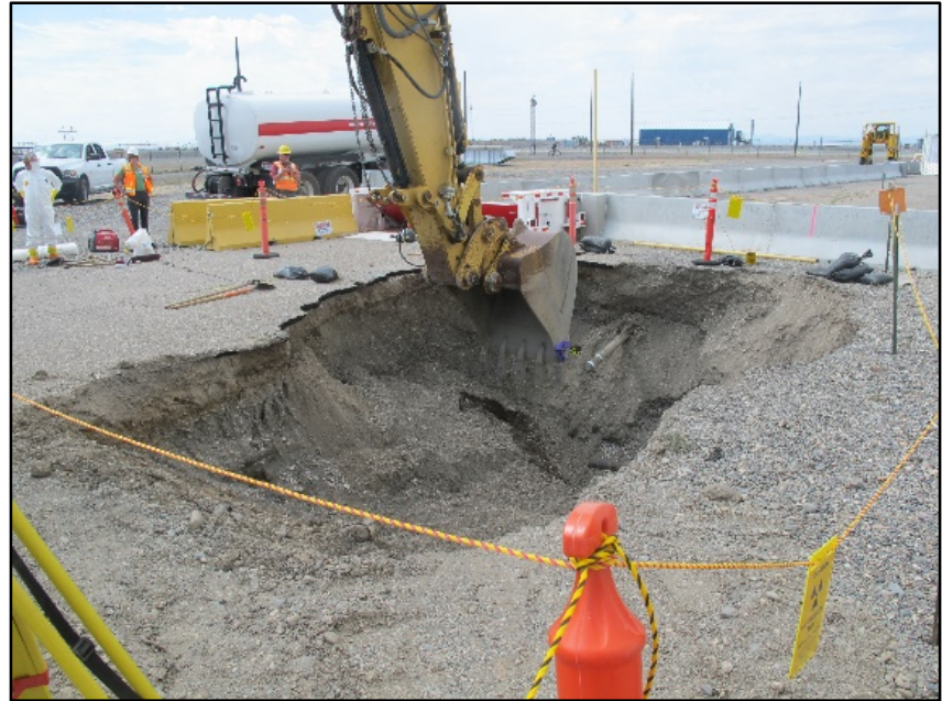
Excavation of CPP-142 Shallow Injection Well
