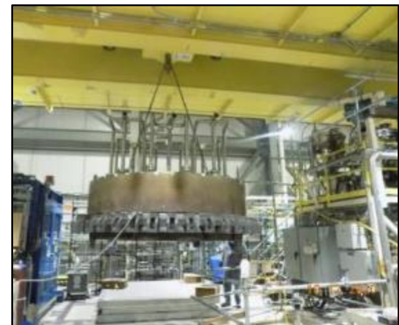
Installing PGF vessel head
