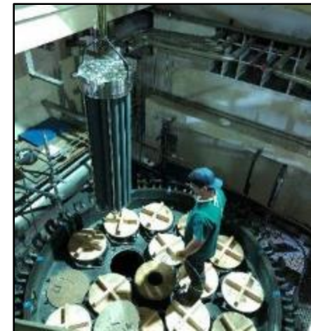
Installing modified PGF bundles
