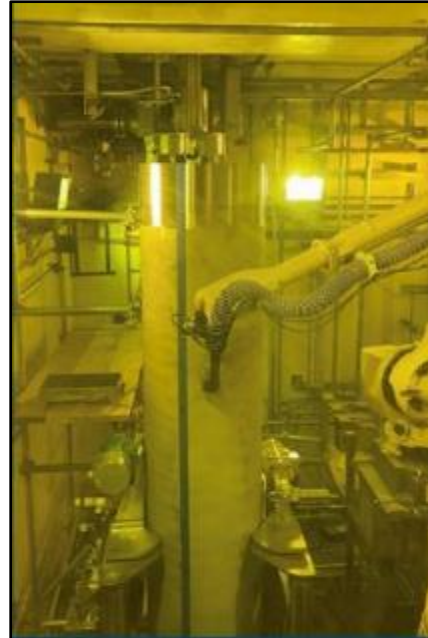
Canister decon robot performing automated decon cycle
