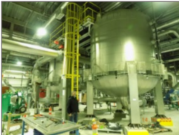
Granular Activated Carbon (GAC) bed vessels
