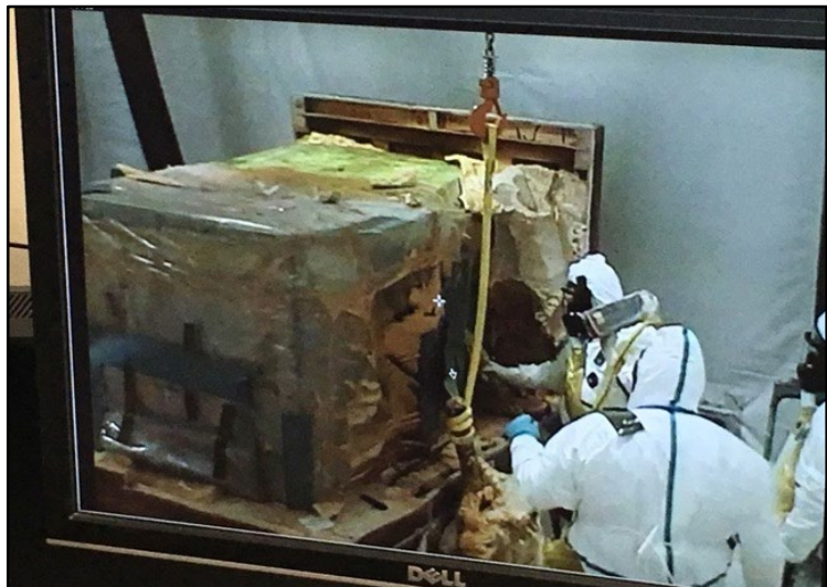
Phased dismantlement of a Mound waste box
