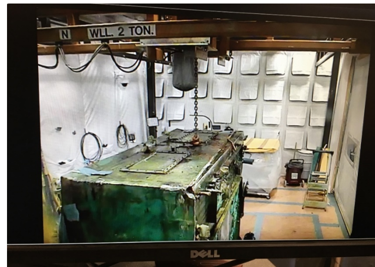
Phased dismantlement of a Mound waste box
