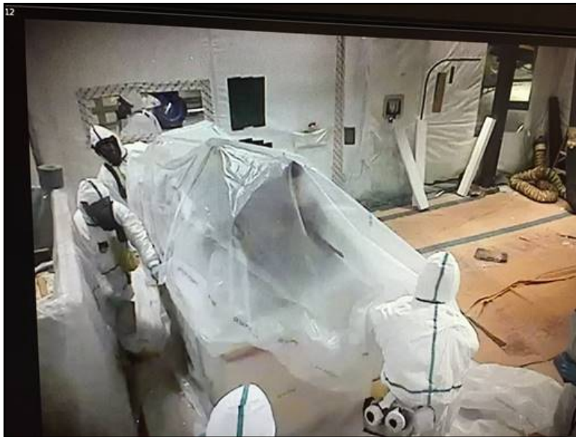
Personnel protective equipment and engineered controls kept workers safe
