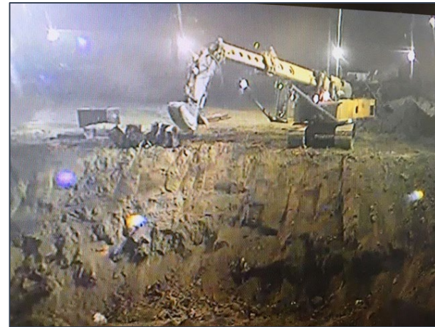
Exhuming targeted buried waste at ARP VIII
