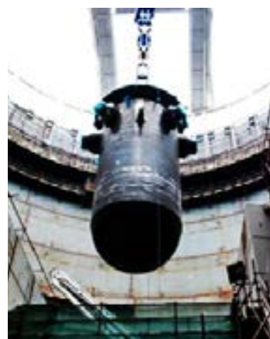
The reactor pressure vessel is cast from solid steel 20 cm (9 inches) thick.
