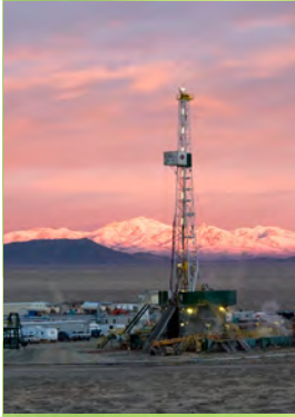
Geothermal drilling at Blue Mountain. Source: GRC
