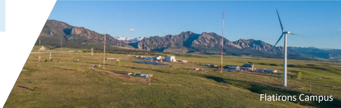
Energy System's Integration Facility
