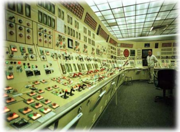
Figure 19. Typical nuclear power plant control room with analog technology.
