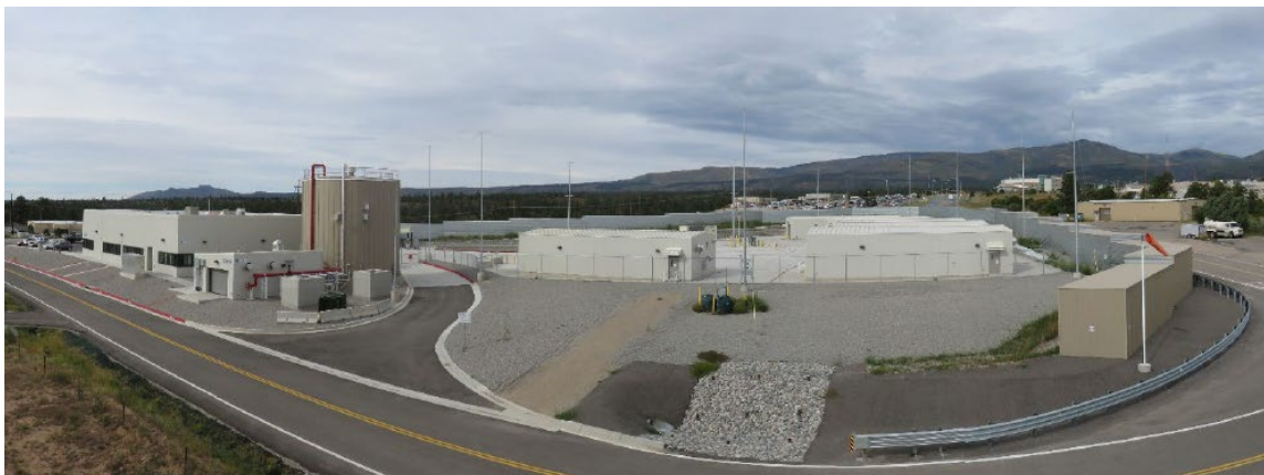
Figure A.4.11-1 TRU Waste Facility at TA-63
