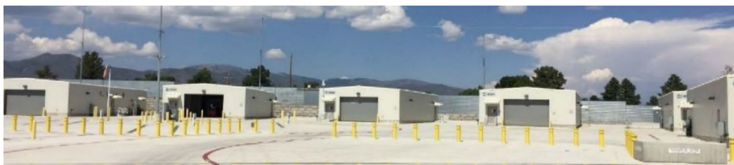
Figure A.2.2-8 Transuranic Waste Facility at LANL
