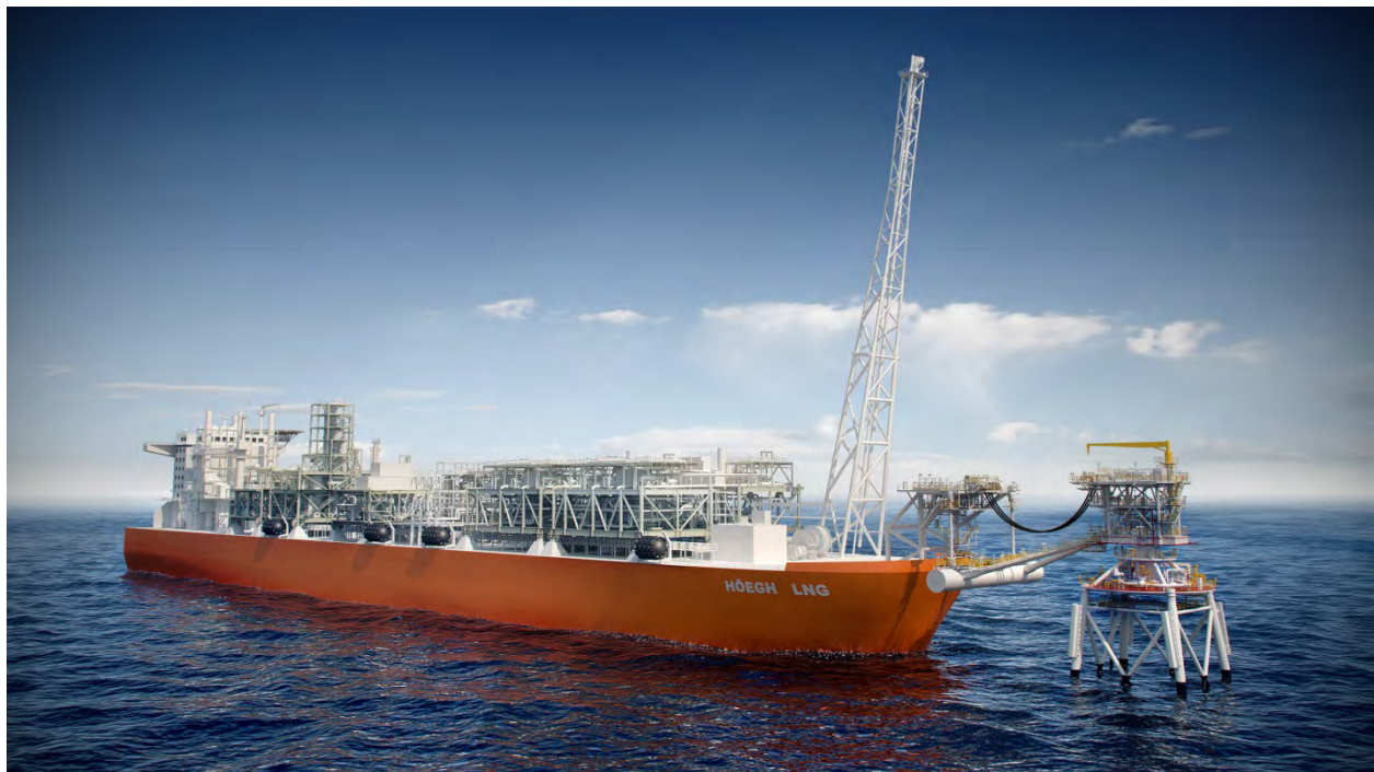
Figure 8 Floating Liquefied Natural Gas Vessel on a Tower Yoke Mooring System
