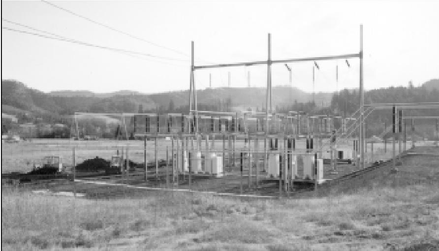
*Substations and electric yards—no vegetation is allowed to grow inside the area, so that electrical “grounding” of equipment and the safety of workers are maintained.*
