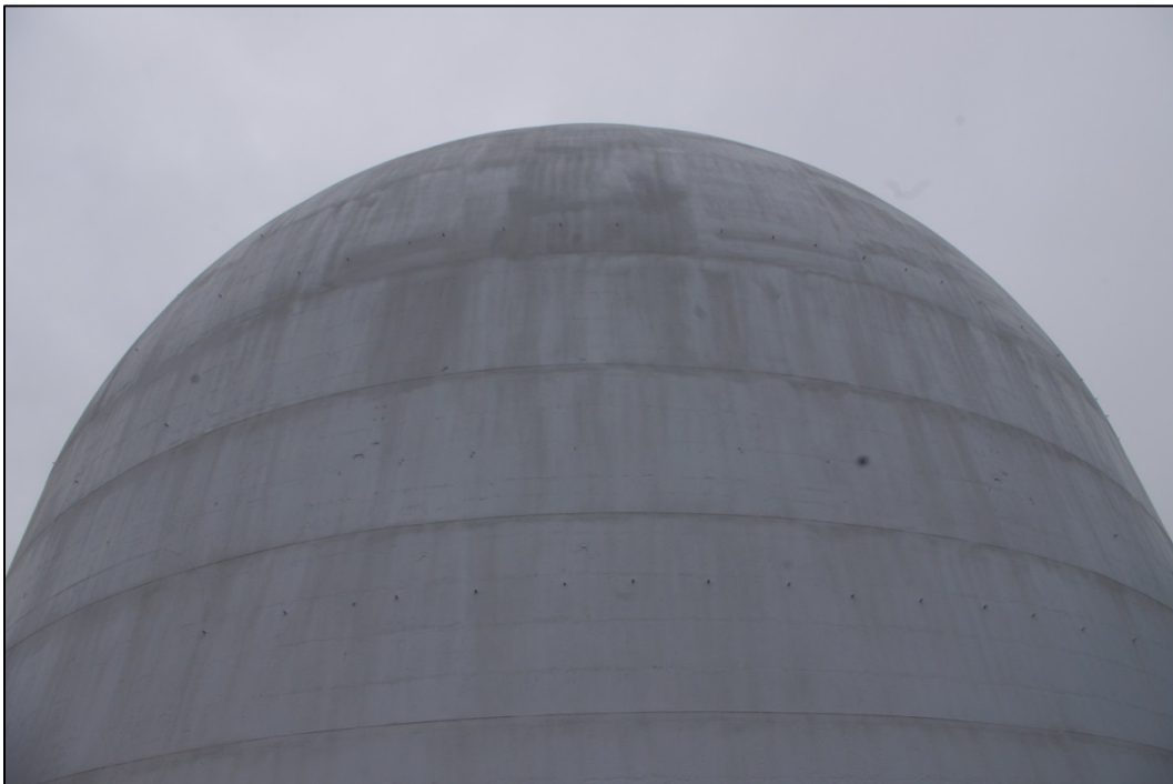
Figure 22. Piqua Reactor Building, Detail View of the Reactor Containment Dome.
