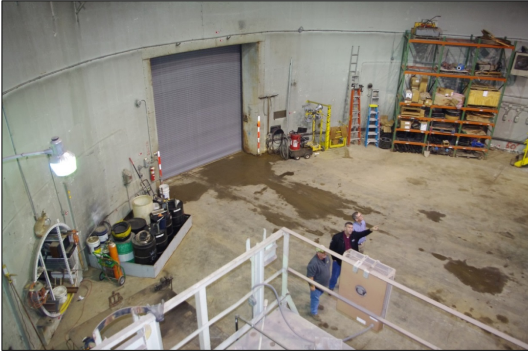
Figure 25. Piqua Reactor Building, Detail View Inside the Concrete Reactor Containment Dome. The reactor was covered by a waterproof membrane and an additional layer of cement after it was defueled during reactor decommissioning.
