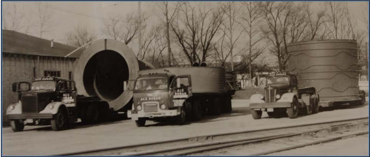
Figure 7. Delivery of the Reactor Vessel.
