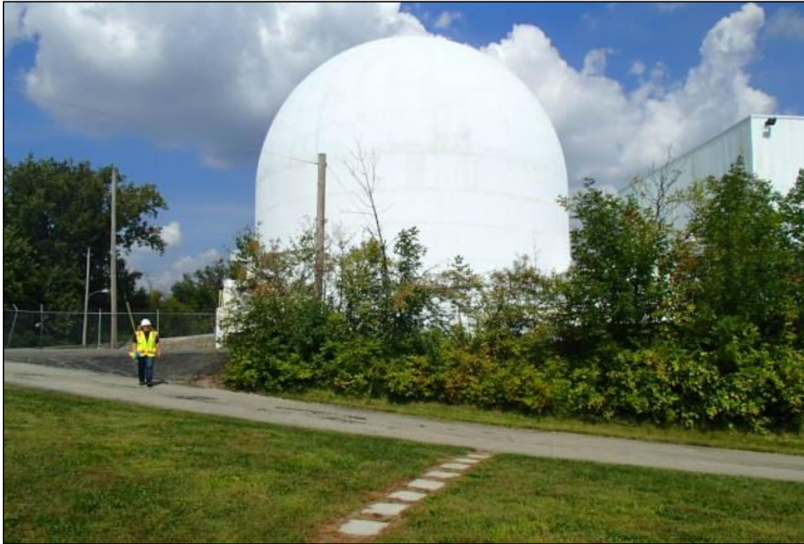
Figure 7: View showing leveled, graded area along southern edge of the APE and sloped terrain immediately to the south, facing north.
