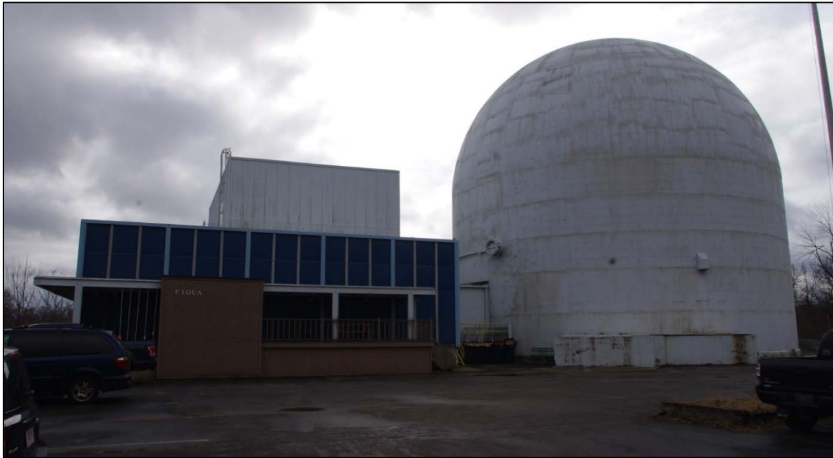
Figure 15. Piqua Reactor Building, Current View, Looking South. The front of the one-story administrative portion is clad in blue panels, the three-story control portion is clad in gray panels, and the reactor containment dome is steel-clad concrete.
