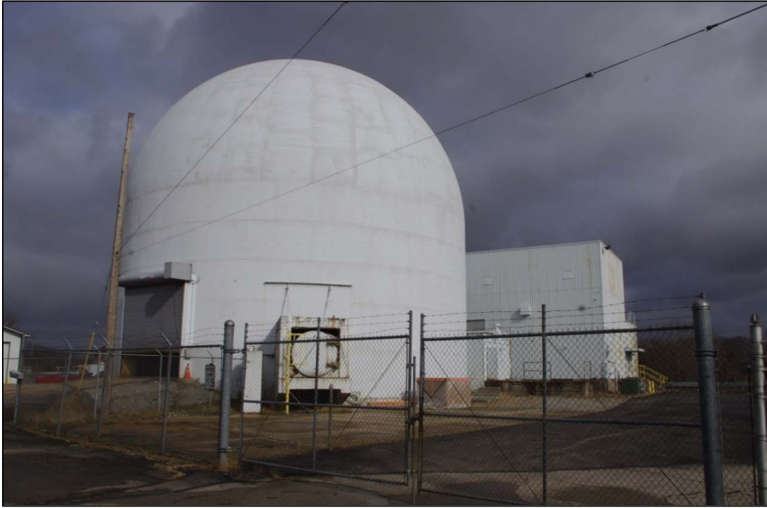
Figure 19. Piqua Reactor Building, Current View, Looking Northeast. The truck access door was cut into the reactor containment dome as part of the reactor deactivation process. The reactor containment dome now provides storage space.
