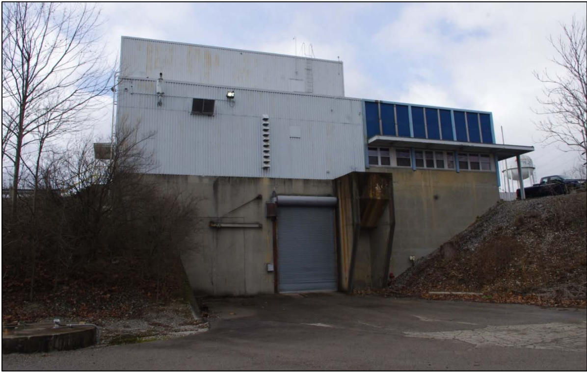
Figure 17. Piqua Reactor Building, Current View, Looking West.
