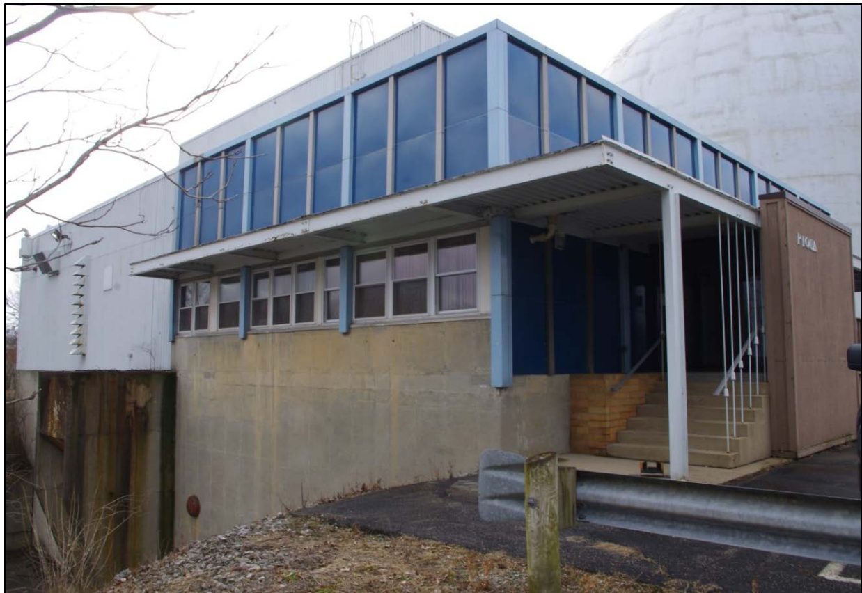
Figure 16. Piqua Reactor Building, Current View, Looking Southwest.
