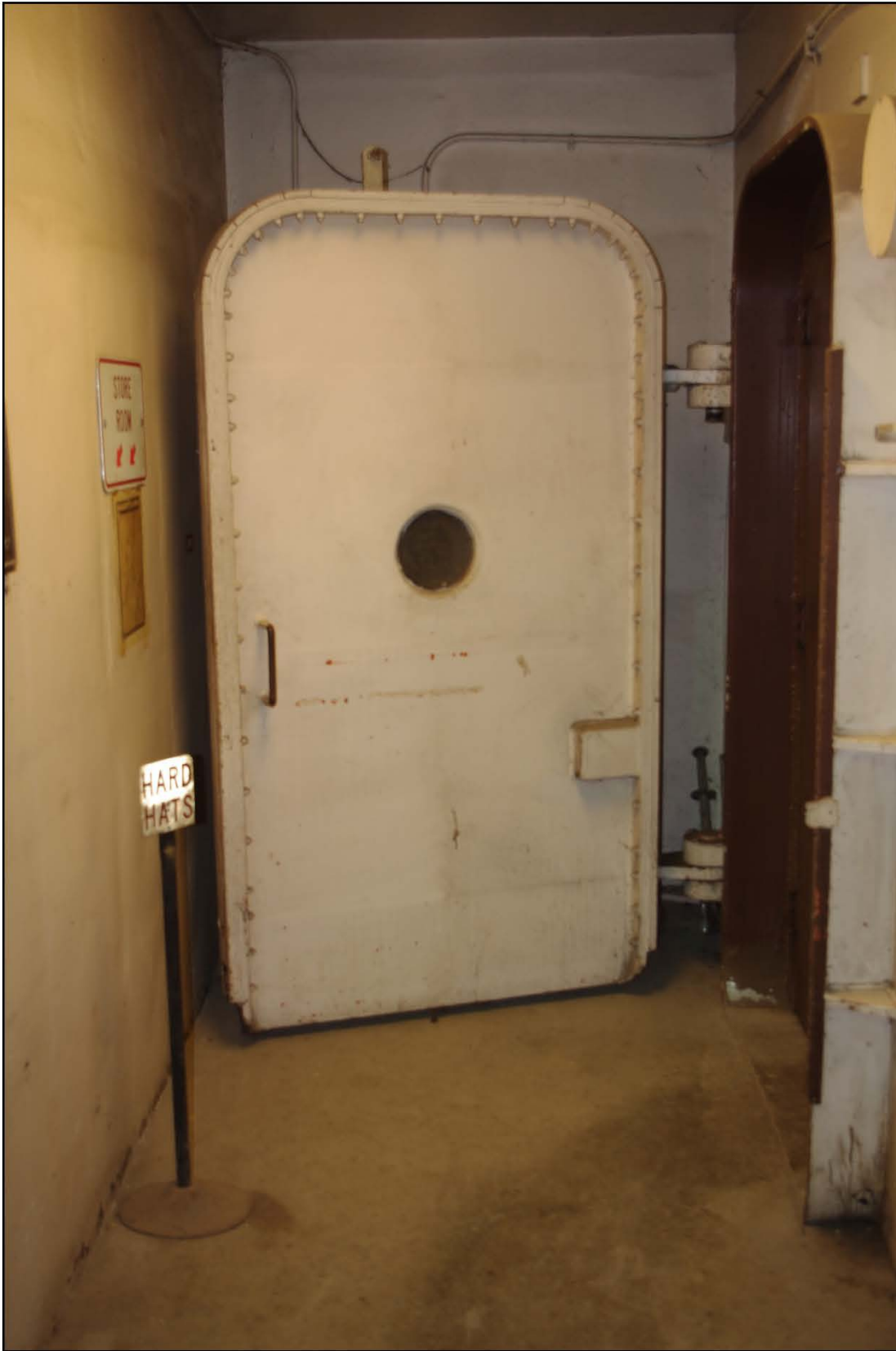
Figure 27. Piqua Reactor Building, Door Detail.
