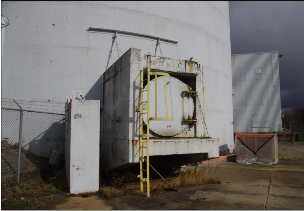
Figure 21. Piqua Reactor Building, Current View.
