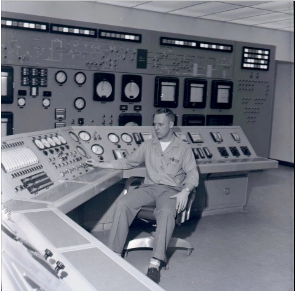
Figure 9. Piqua Reactor Building Control Room, Circa 1962.
