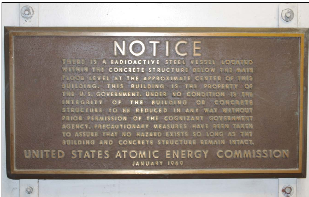
Figure 29. Piqua Reactor Building, Detail of Placard. This is one of three identical placards that provide legacy information about the reactor vessel that is entombed inside the concrete containment dome.
