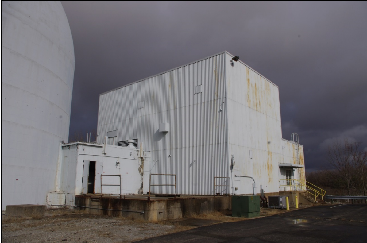
Figure 18. Piqua Reactor Building, Current View, Looking Northeast.
