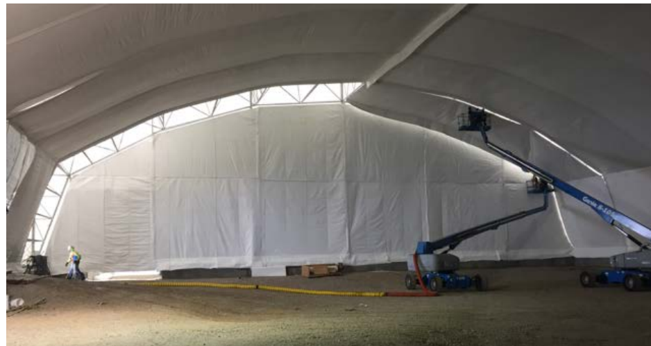
ARP IX Retrieval Enclosure – near completion of inner liner installation.
