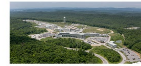
Spallation Neutron Source (SNS) OAK RIDGE NATIONAL LABORATORY
