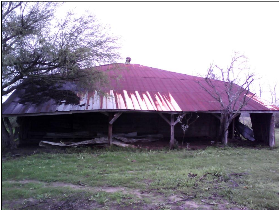
Figure 5.7 Historic standing structure HSS-FB-2 looking northeast
