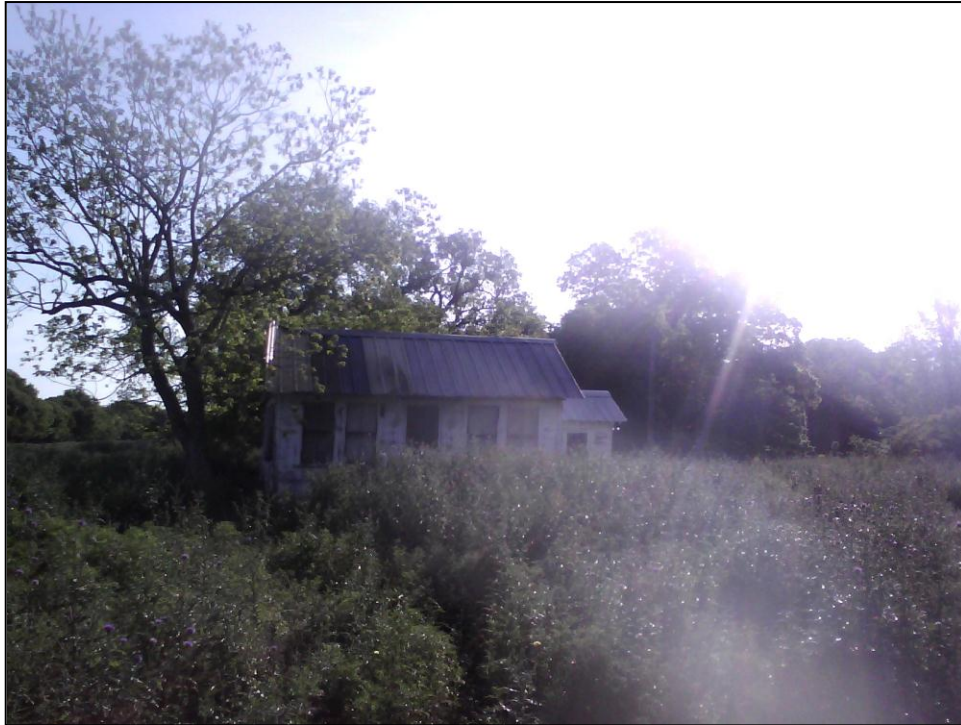
Figure 5.22 Historic standing structure HSS-WH-1 looking east
