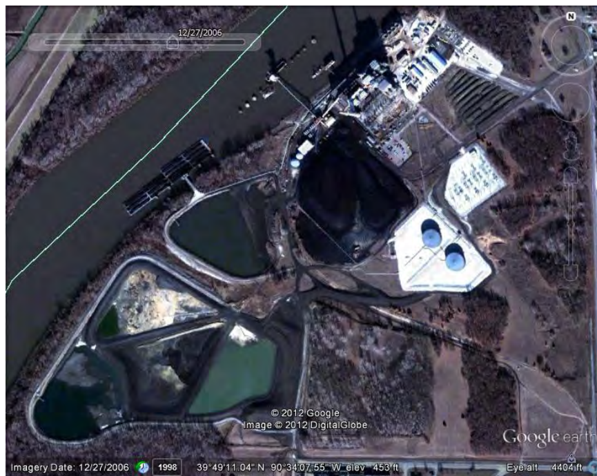
Photo #4 Meredosia Energy Center 2006 Google Earth 2012
