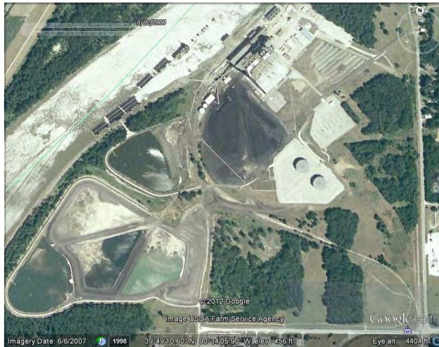
Photo #3 Meredosia Energy Center 2007 Google Earth 2012
