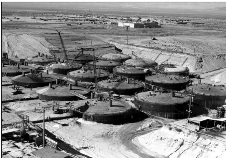
**Figure 2–1. Single-Shell Tanks Under Construction at the Hanford Site, 1947–1948**
