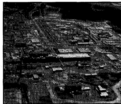
Savannah River Site.
