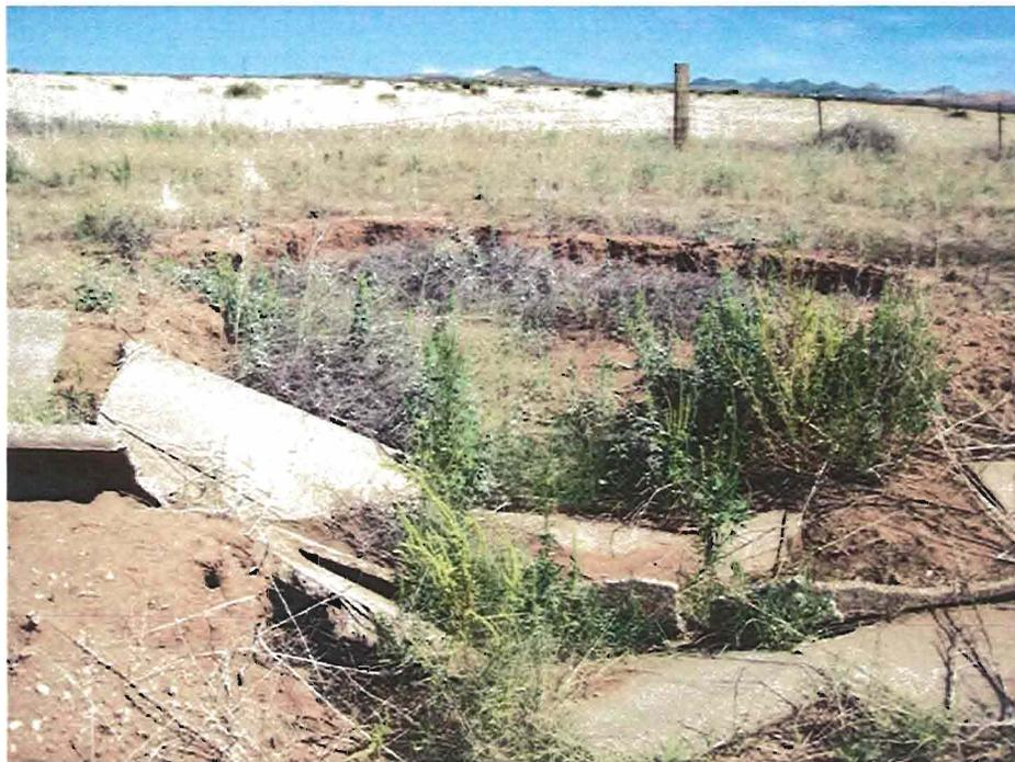
Photograph 13 – Eroded drainage feature at break in irrigation ditch (September)
