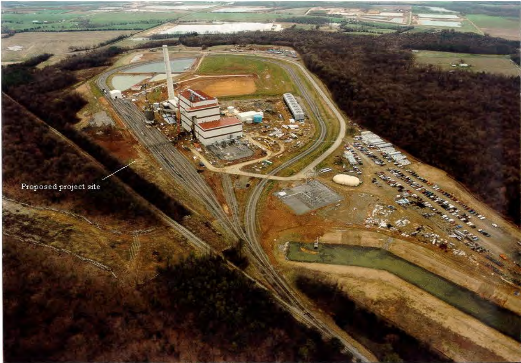
Figure 3. Aerial photograph of Mirant-Birchwood Power Plant taken April 10, 1996.
