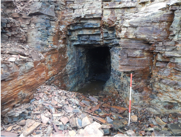
Example Adit: A mine opening greater than 10 feet deep driven horizontally for the purpose of providing access to a mineral deposit. A portal is a surface entrance to an adit.
