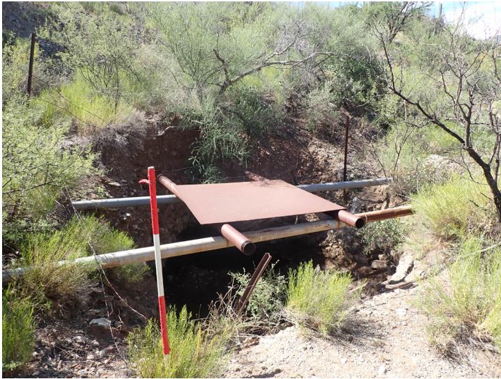
Example Shafts: Vertical openings that lead to an underground mine.
