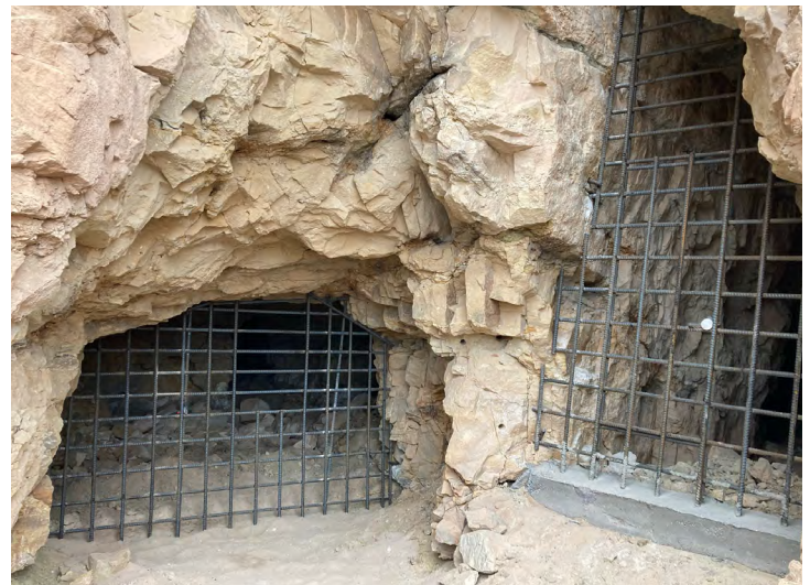
Adit at the Mucho Claims Mine, located southeast of Green River, Utah, before and after safeguarding (BLM-administered land).
