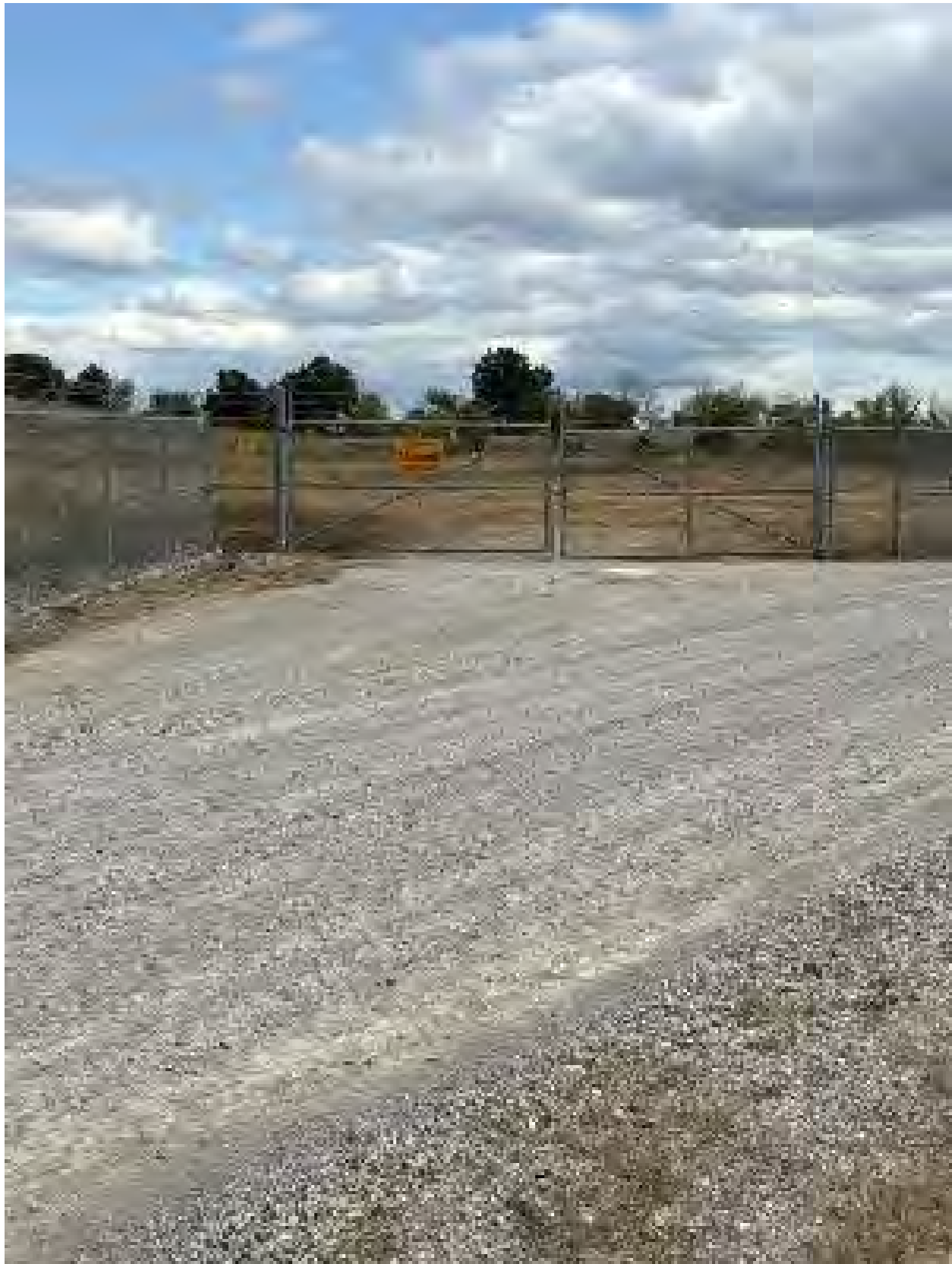
OSDF South Gate, North-Northeast Perspective
