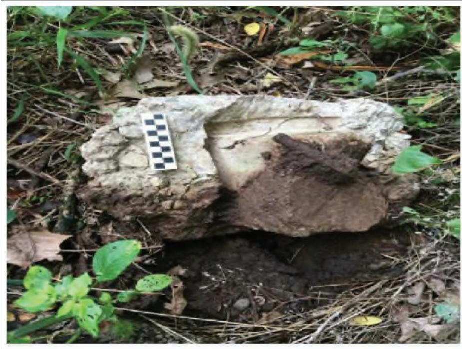
Figure 36. Close-up of Concrete Fencepost Remnant
