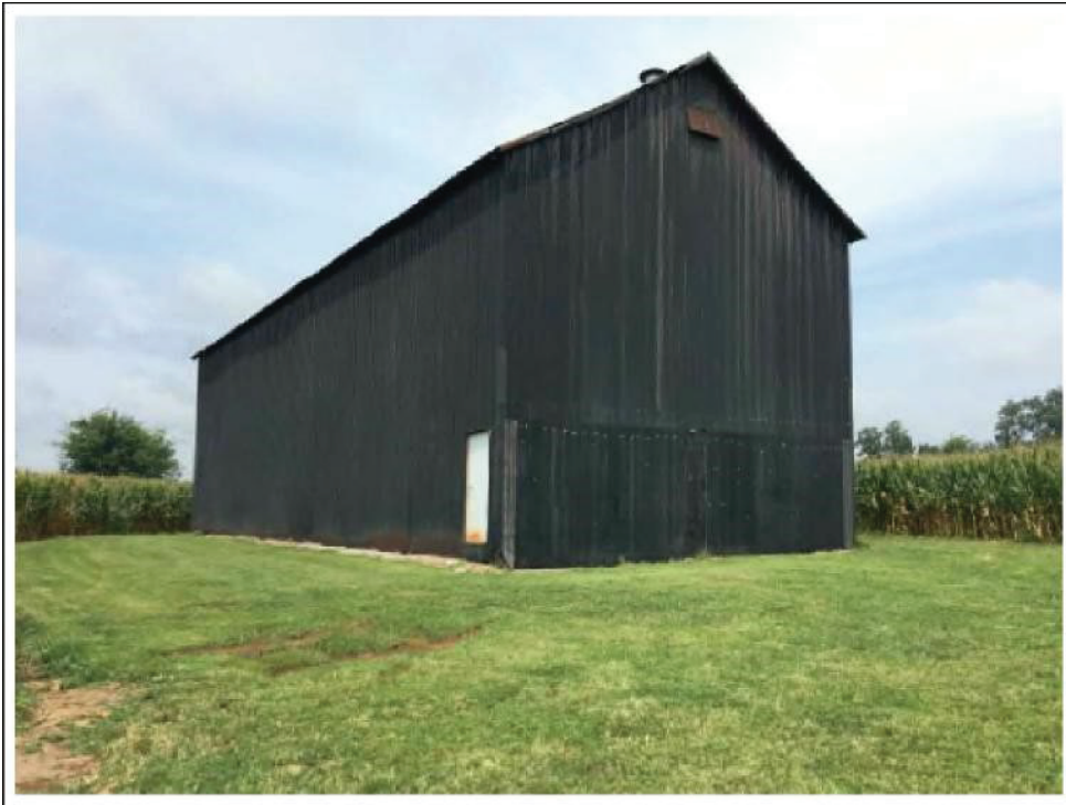
Figure 27. Northwest Facing H-1 Barn
