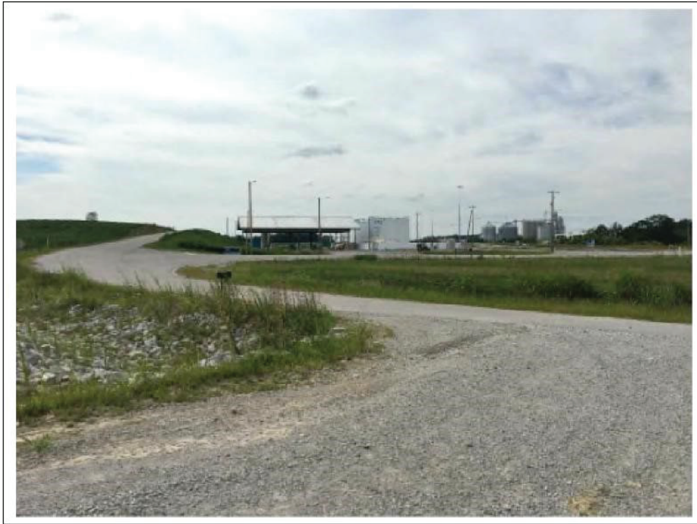
Figure 10. Southwest Facing CSX Facility
