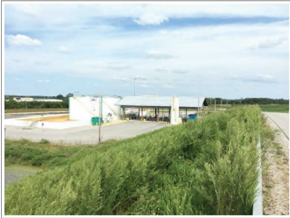
Figure 9. Northeast Facing CSX Facility
