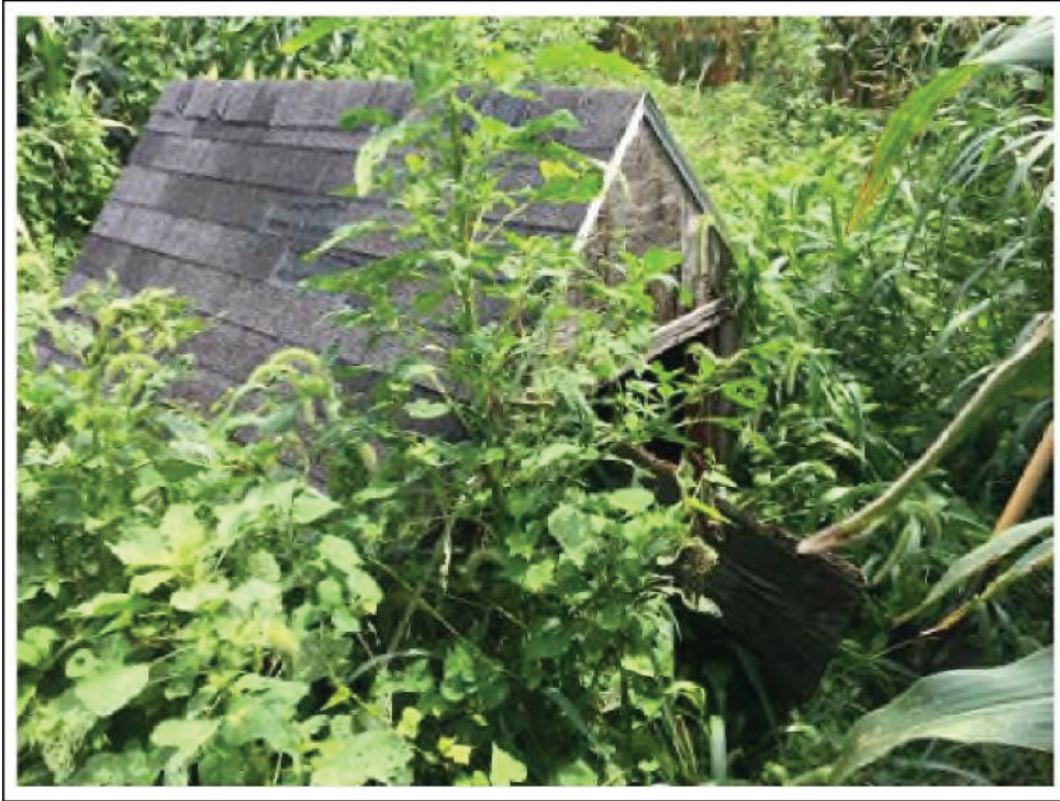
Figure 28. East Facing H-1 Pumphouse
