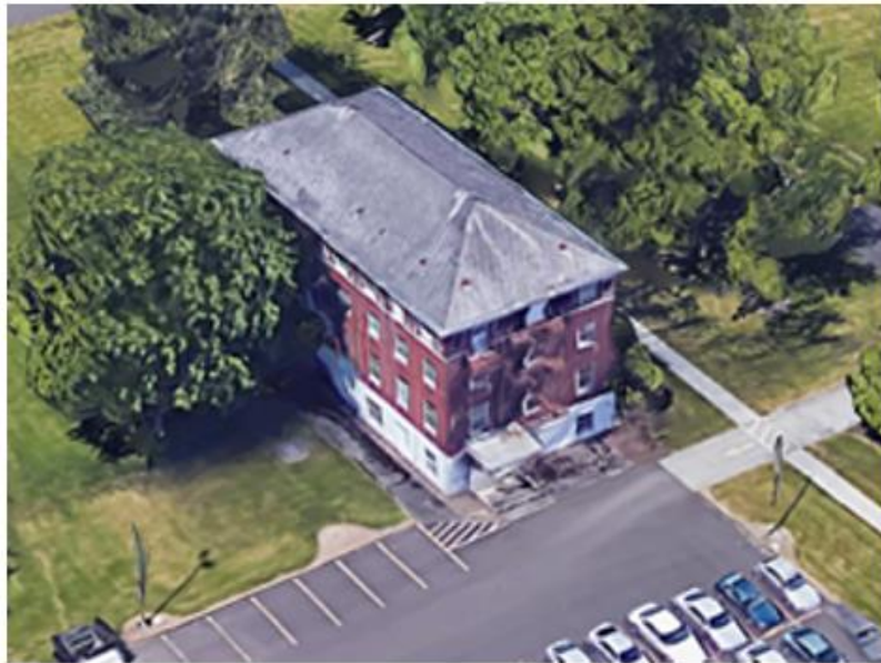
★ Building 2: Looking Northeast
