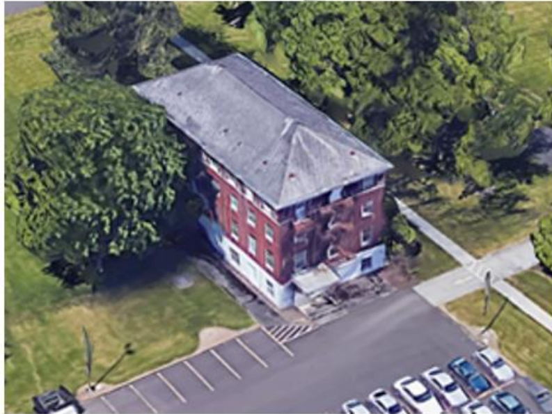
★ Building 2: Looking Northeast
