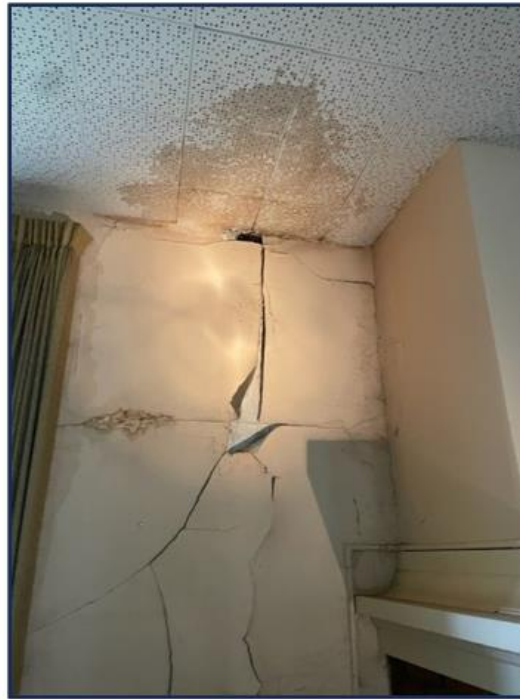
Examples of chronic water damage evidence and suspected mold identified throughout B-2 Basement
