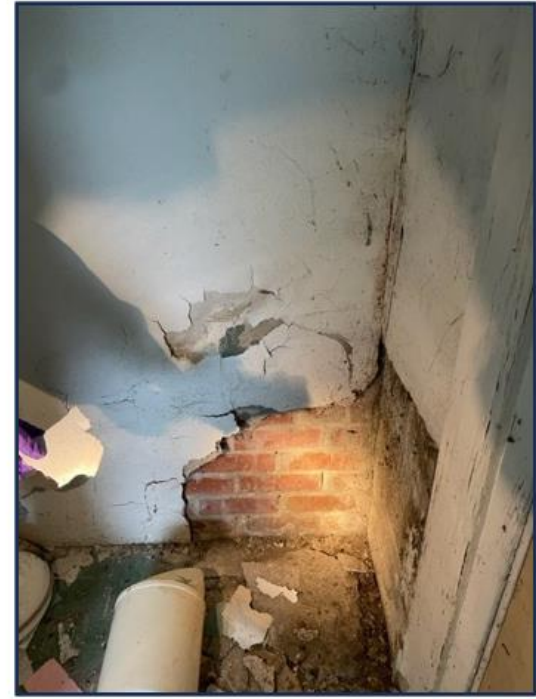
Examples of chronic water damage evidence and suspected mold identified throughout B-2 Basement
