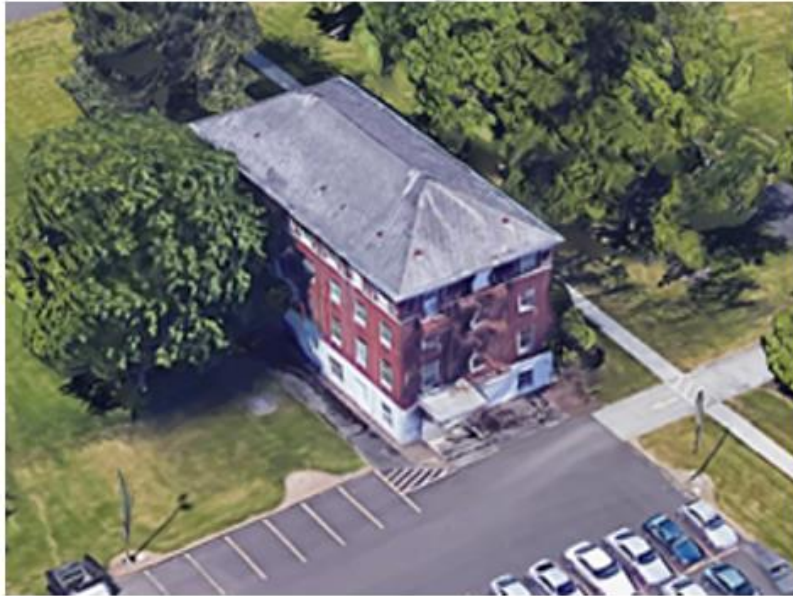
★ Building 2: Looking Northeast
