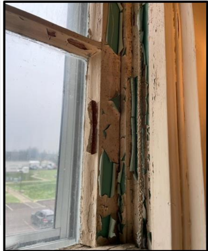
Interior paint on window (Room 302) exhibiting multiple layers of historic paint
