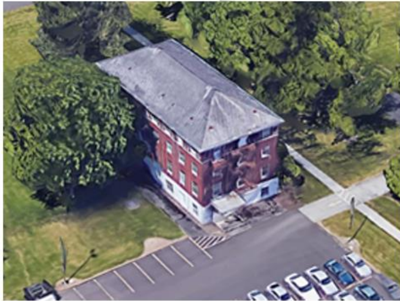
★ Building 2: Looking Northeast
