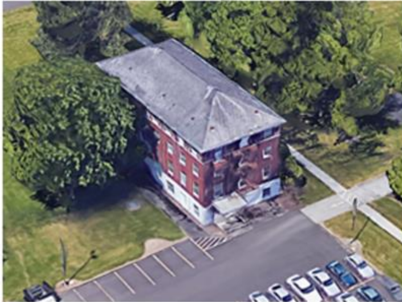
★ Building 2: Looking Northeast
