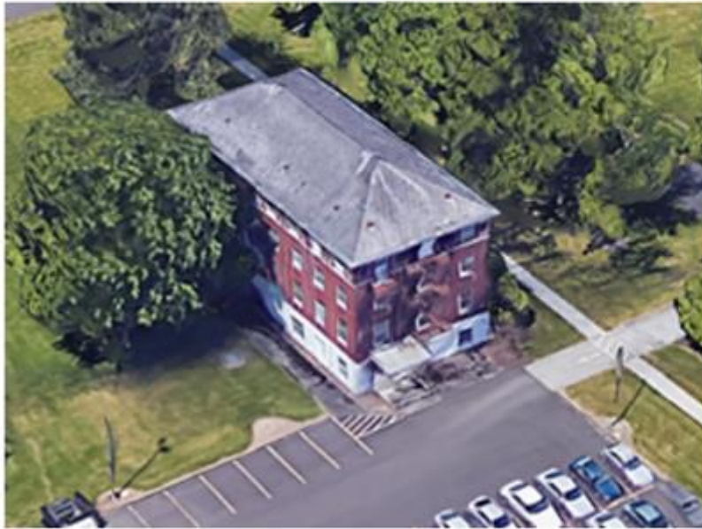
★ Building 2: Looking Northeast
