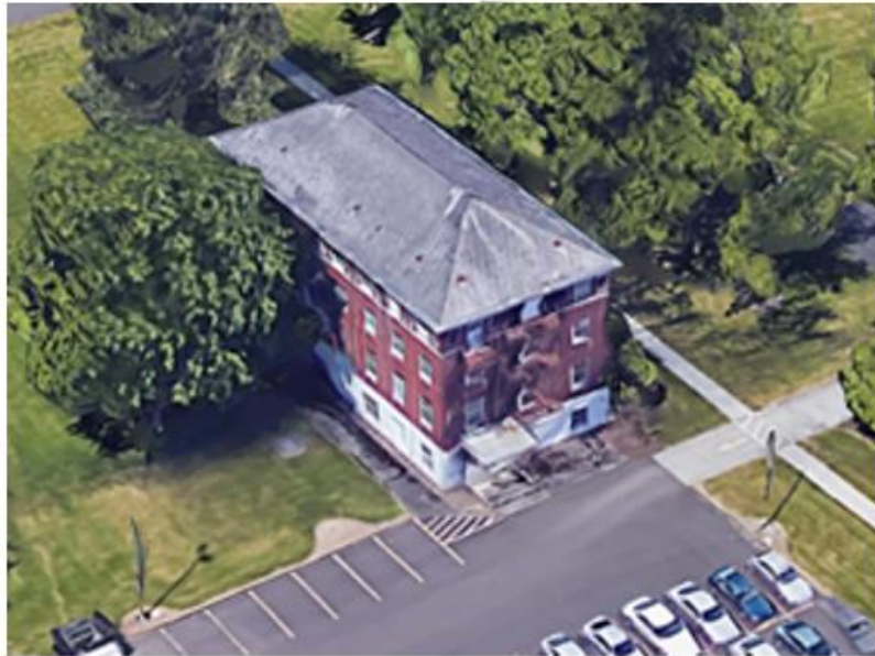
★ Building 2: Looking Northeast
