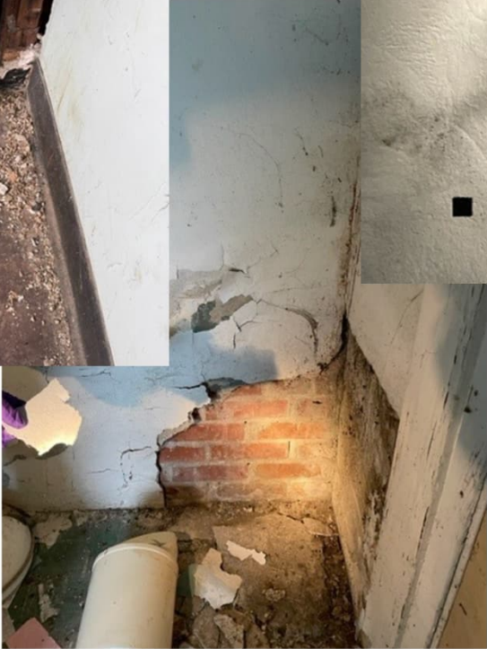
Examples of significant water damage and decay
