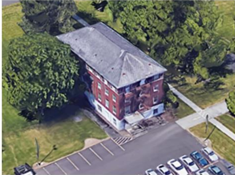
★ Building 2: Looking Northeast
