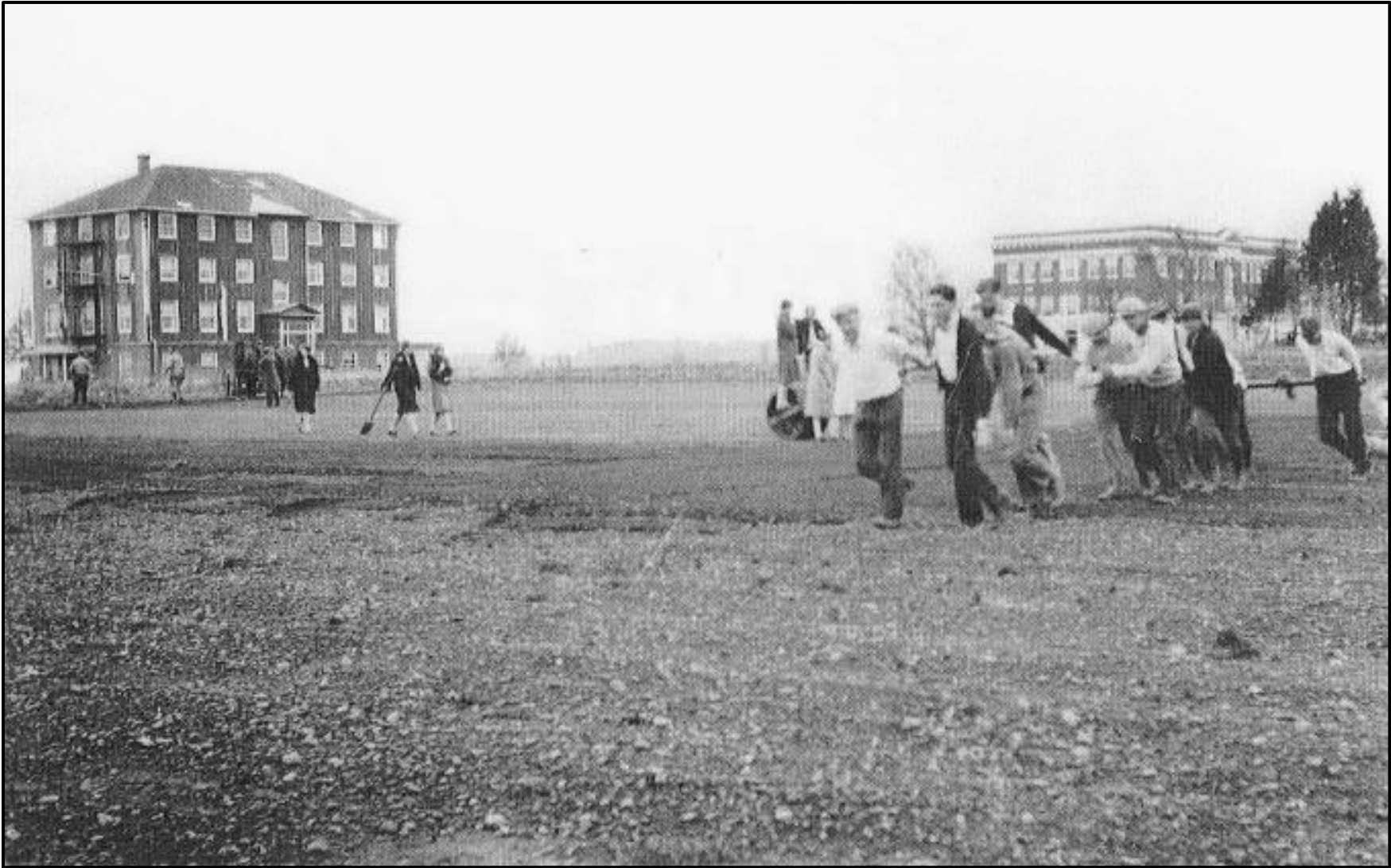
1 2 Source: An Evaluation of the Historic Significance of the Department of the Interior, Bureau of Mines, Northwest Electrodevelopment Laboratory/ 3 ARC, Albany, Oregon (Vol. 1) 4 Figure 2-2: B-2 Building Exterior Post-1926 (Looking Northwest)
