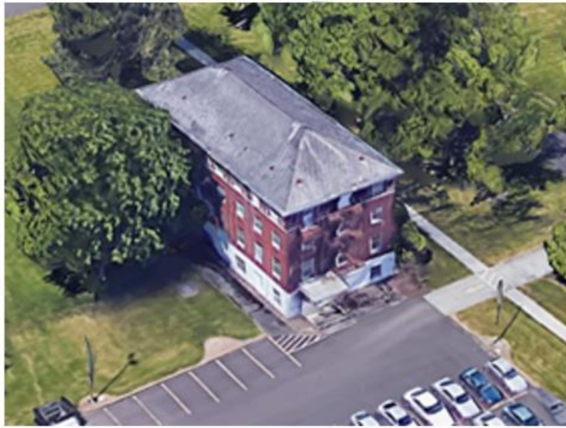
★ Building 2: Looking Northeast
