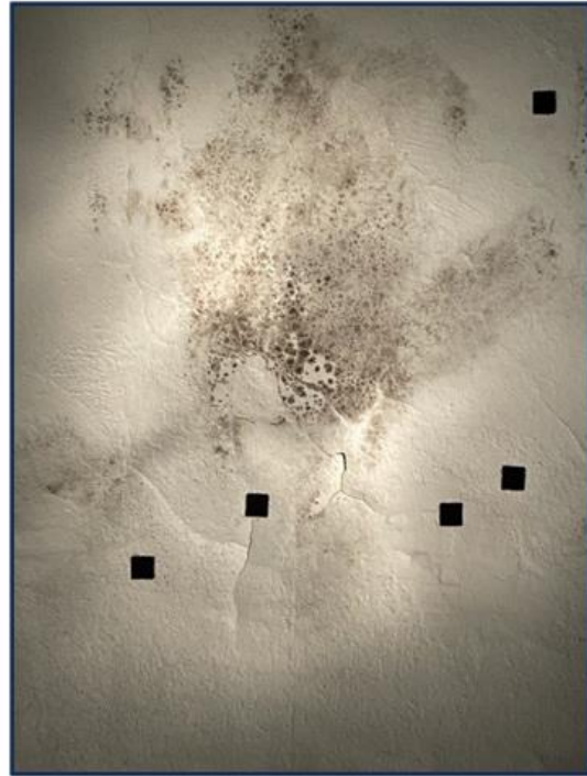
Examples of chronic water damage evidence and suspected mold identified throughout B-2 Basement
