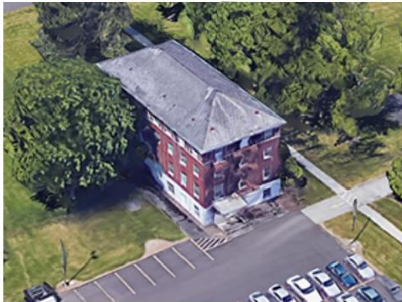
★ Building 2: Looking Northeast
