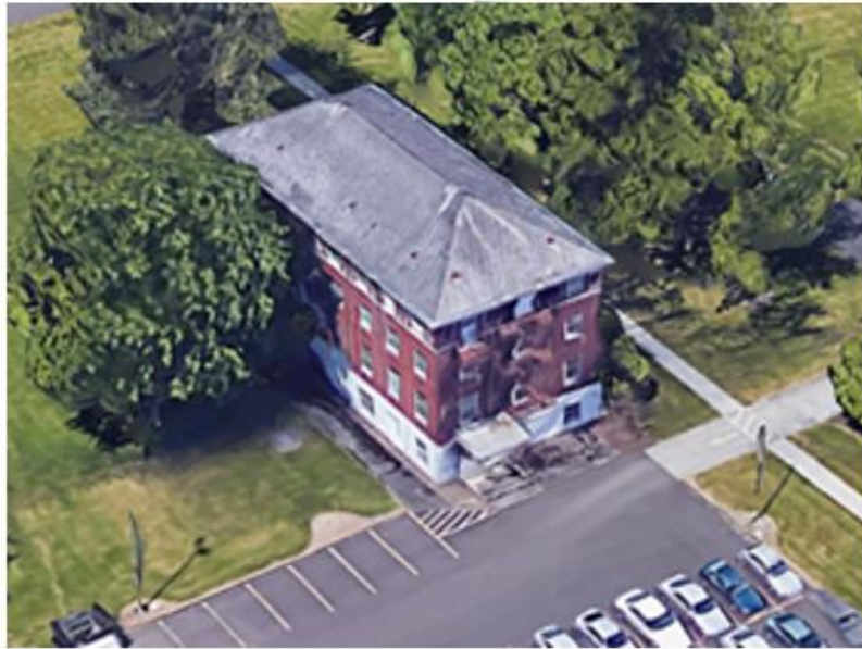
★ Building 2: Looking Northeast
