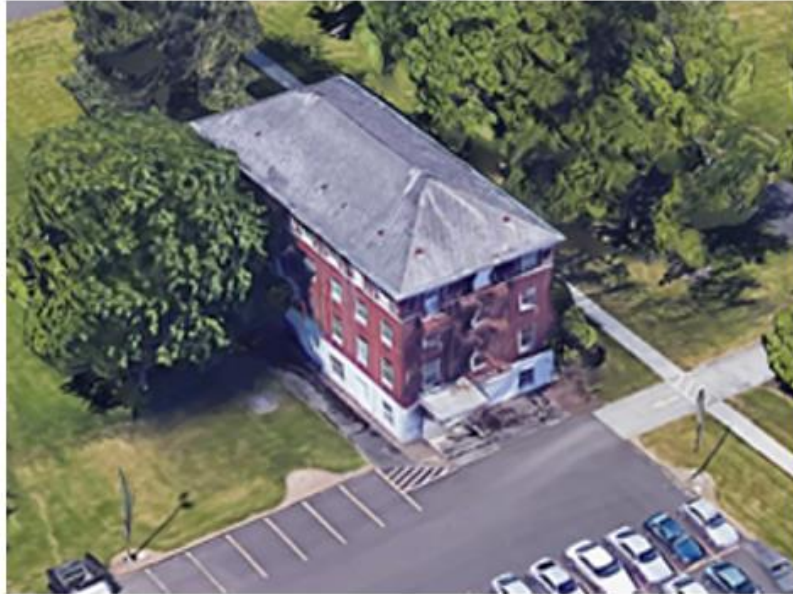
★ Building 2: Looking Northeast
