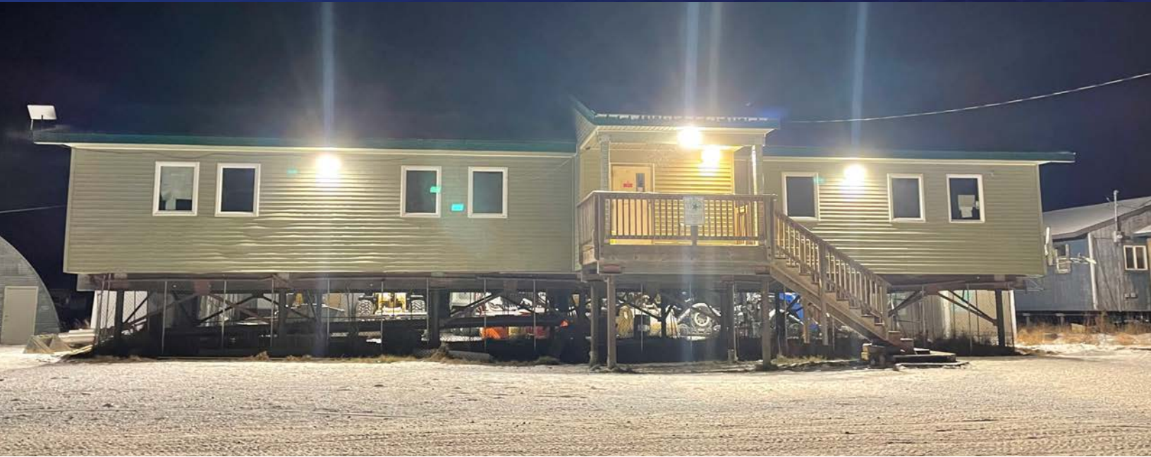
The Tribal Office building in Akiachak. Image by N. George/ANC.
