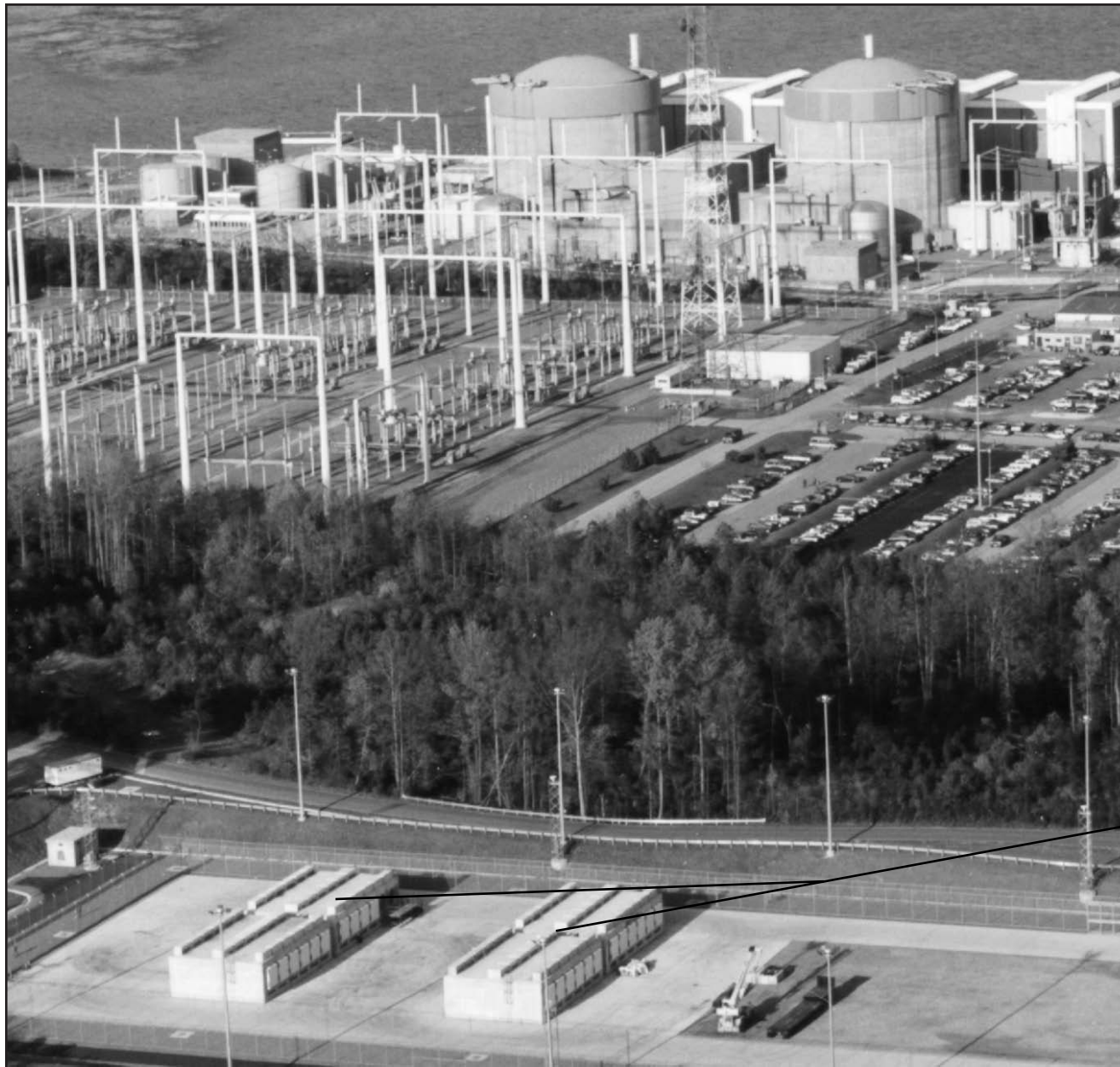
Figure 2-32. Typical independent spent fuel storage installation.
