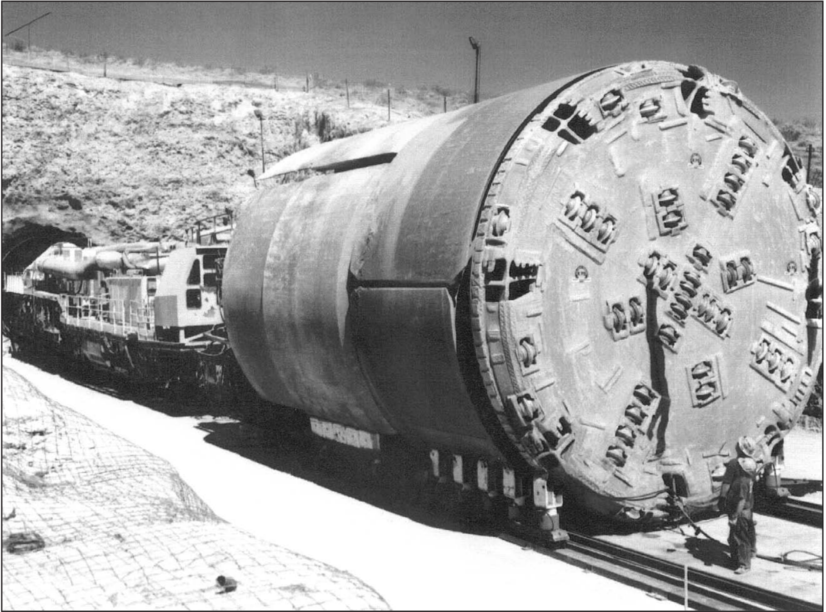
Figure 2-14. Tunnel boring machine.
