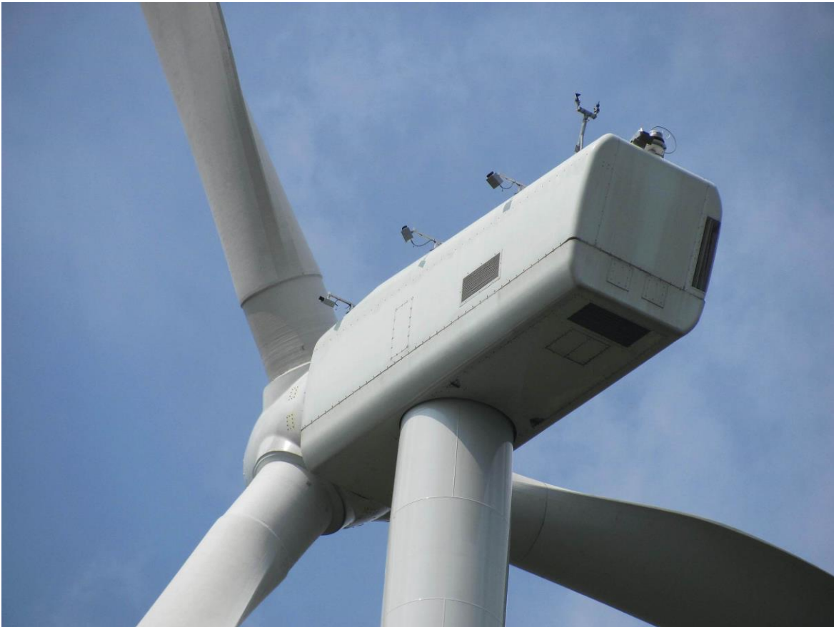
Ultrasonic acoustic deterrents mounted on the side of the nacelle (photo by E. B. Arnett)
