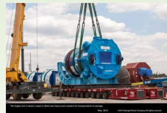
Placement of CVBH on the Unit 4 Nuclear Island and arrival of Unit 4 reactor vessel (Courtesy of Georgia Power/Southern Company)
