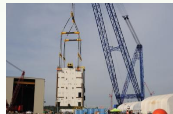
VC Summer Unit 2 CA20 module being removed from module assembly building and set in place (Courtesy of SCANA)
