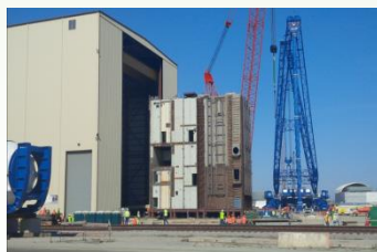
VC Summer Unit 2 CA20 module being removed from module assembly building and set in place (Courtesy of SCANA)
