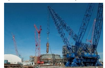
SCE&G Places Final Unit 2 Containment Vessel Ring; The First U.S. AP1000 Steam Generator is placed in Unit 2(Courtesy of SCE&G)
