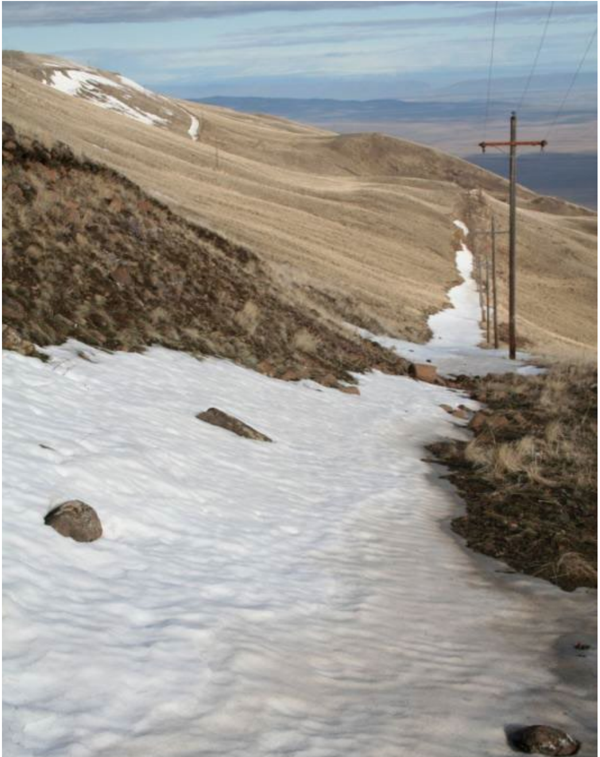
Figure 8 – Benton PUD Overhead Electrical Power and Fiber Optic Telecommunication Poles and Cables (Locale 9A) on Rattlesnake Mountain (Source: DOE/EA-1660F)
