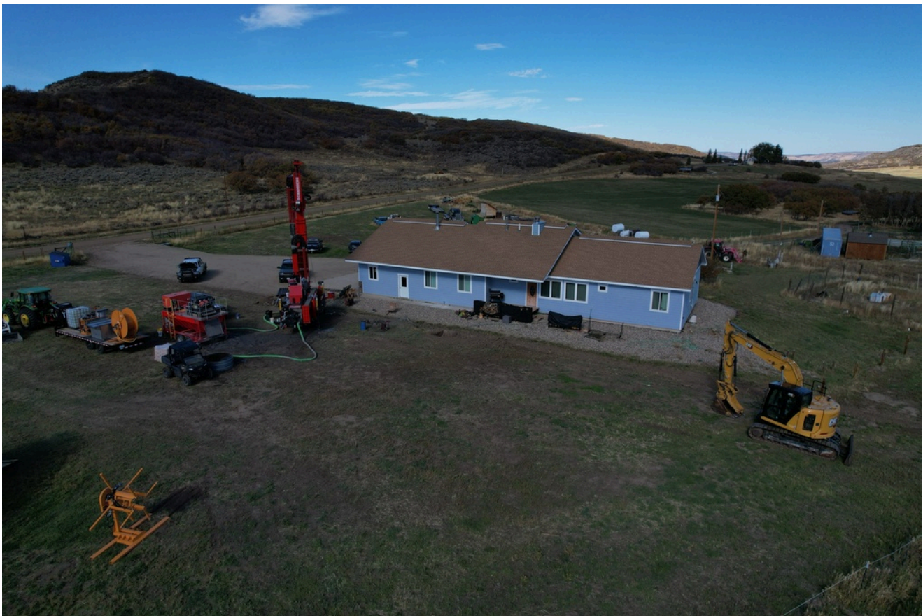
A drill sits outside the Cooper family ranch as they work to install a geothermal heat pump Thursday, Oct. 9, 2025, in Hamilton, Colo. (AP Photo/Brittany Peterson)
