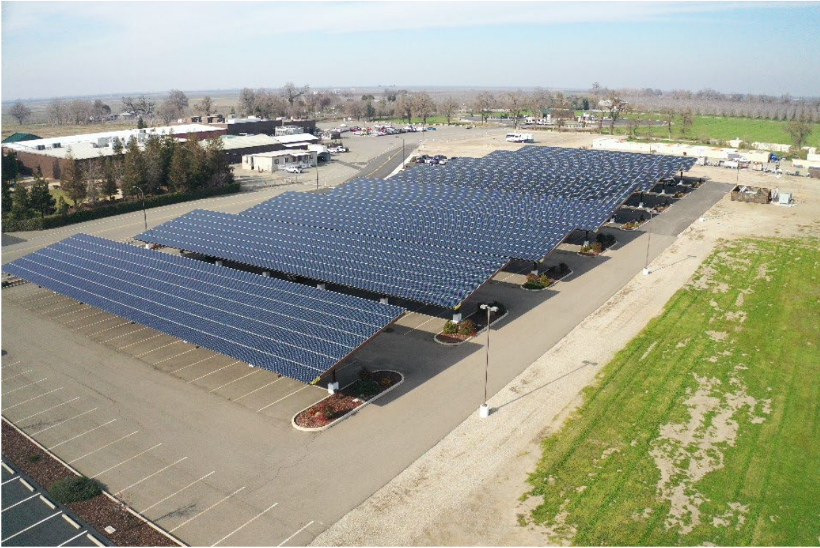
Image 4: Completed canopy construction
