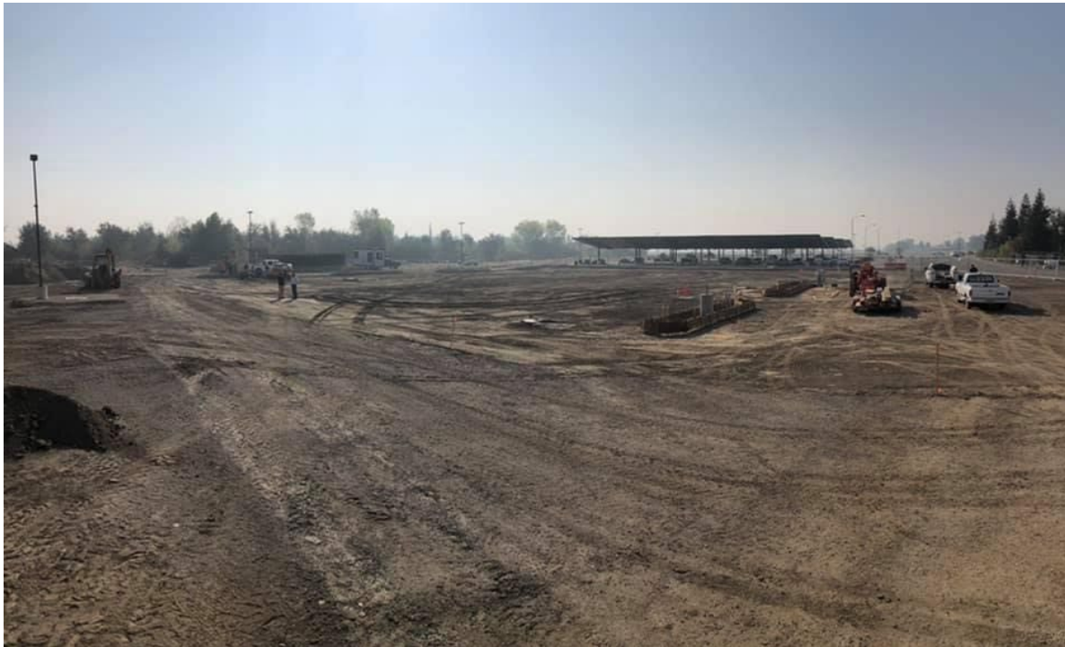
Image 1: Initial construction phase
