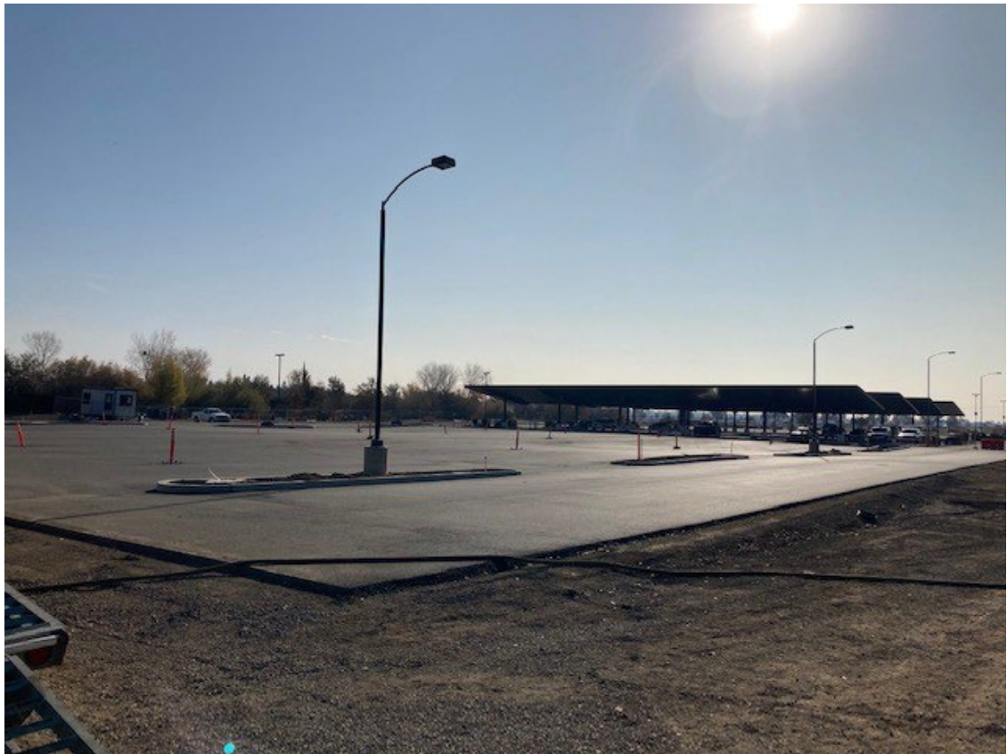
Image 3: Paving complete before canopies were erected
