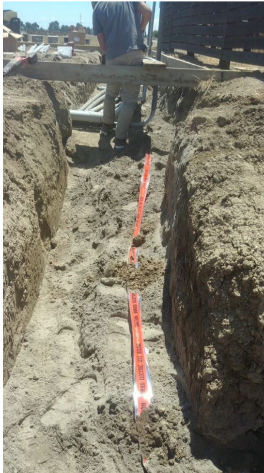
Image 3: Underground medium-voltage cable trenching
