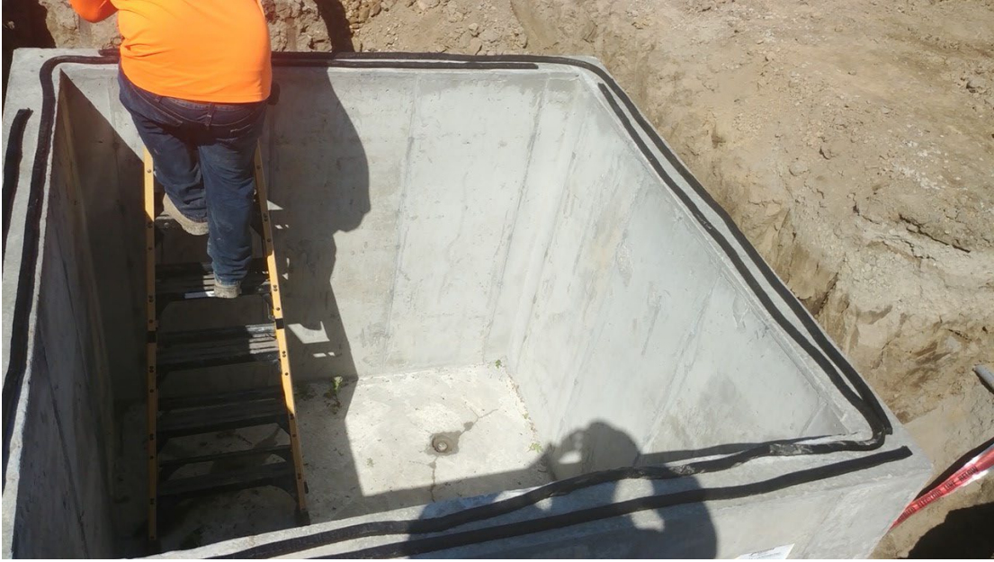
Image 2: One of several new underground electrical vaults
