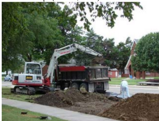
Figure 7.1.15-3: Removal of Contaminated Soil from a Schoolyard in Iola
