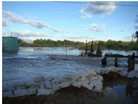
Figure 18.1.15-4: Iowa Avenue in Hudson, WY Under Water
