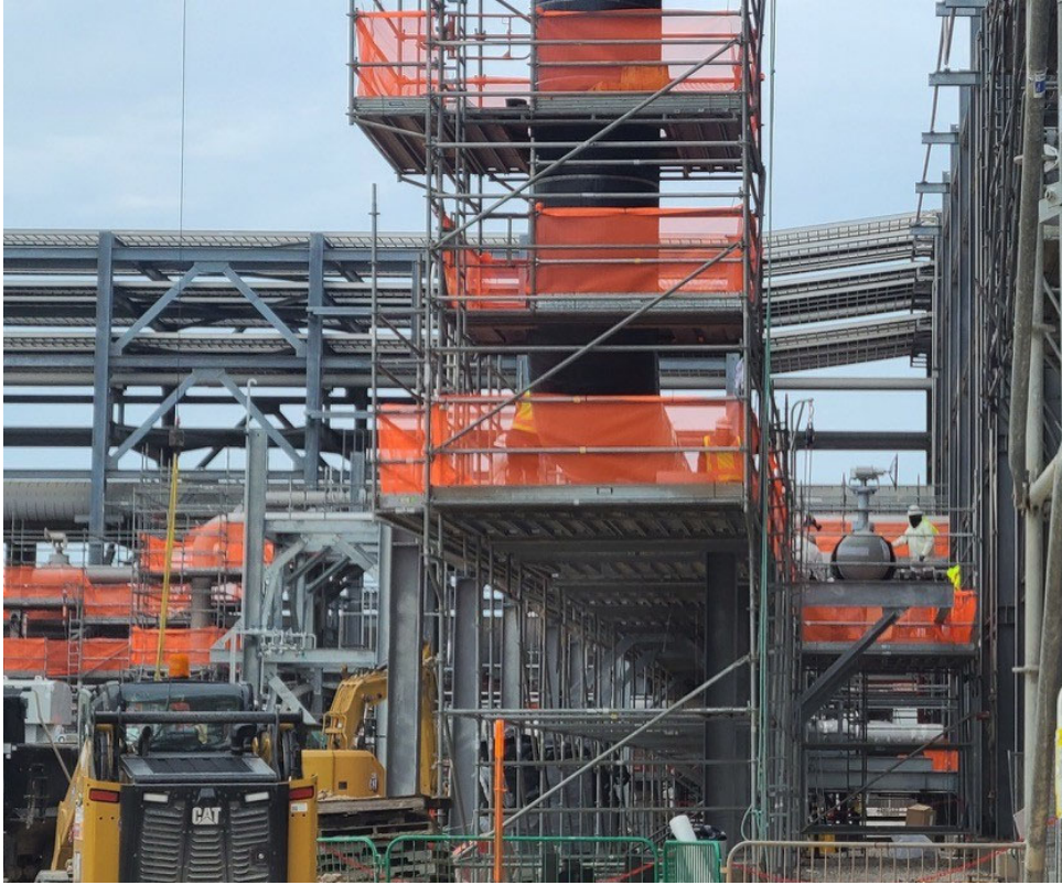
Photo 3: BOG 6 Pipe Insulation
