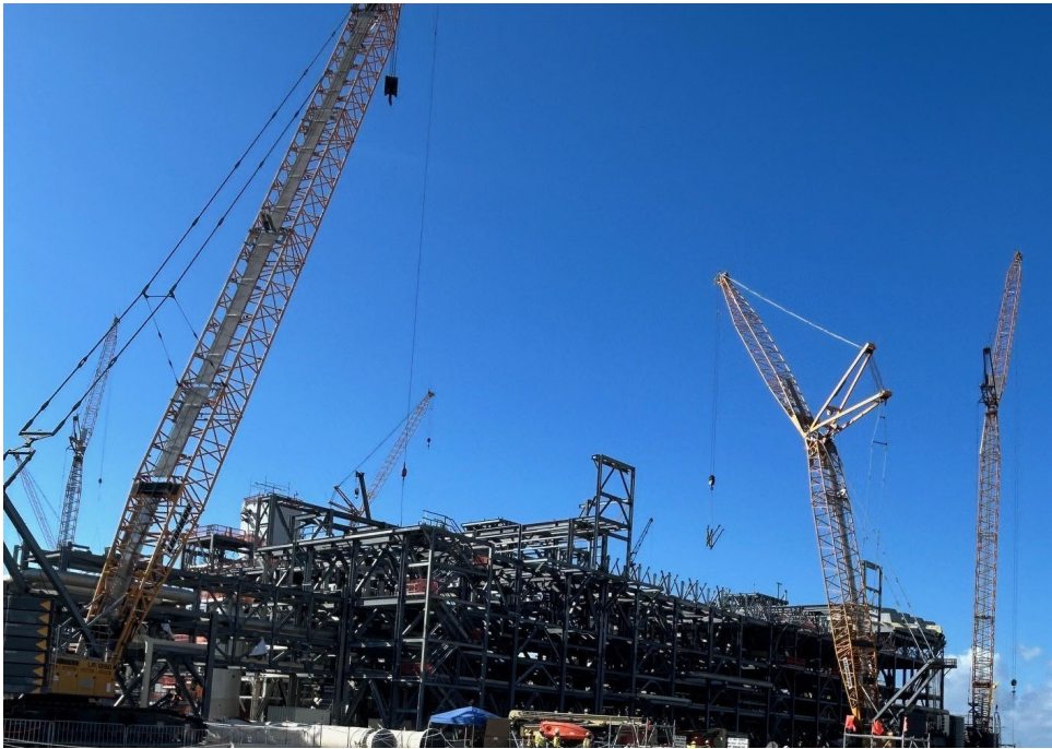
Photo 2: Train 7 Structural Steel Installation
