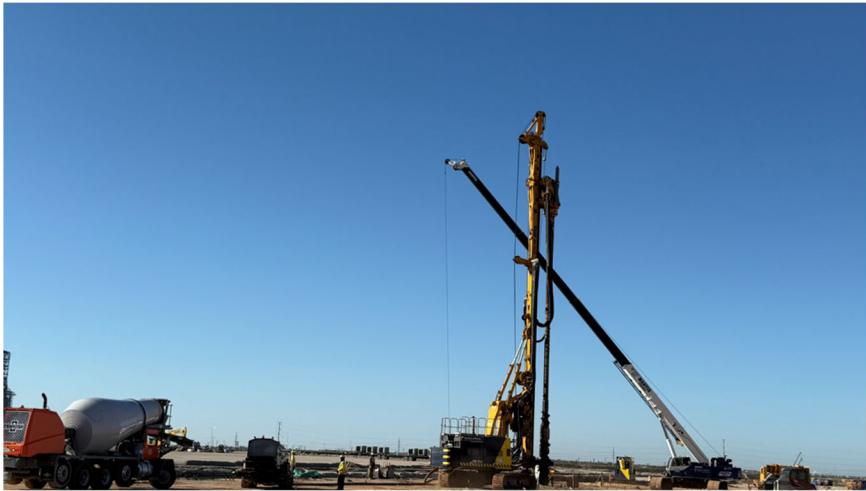
Photo 4: Train 9 Pile Installation
