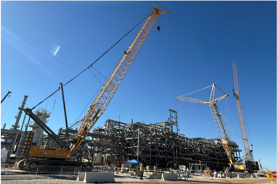
Photo 2: Train 7 Structural Steel
