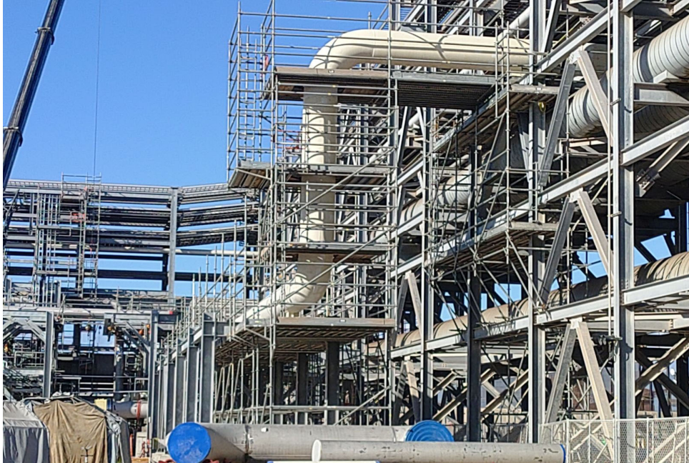
Photo 3: BOG 6 Pipe Installation
