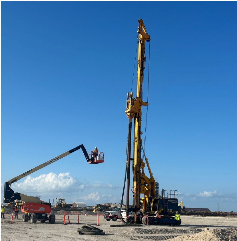
Photo 5: Train 8 Piling Rig
