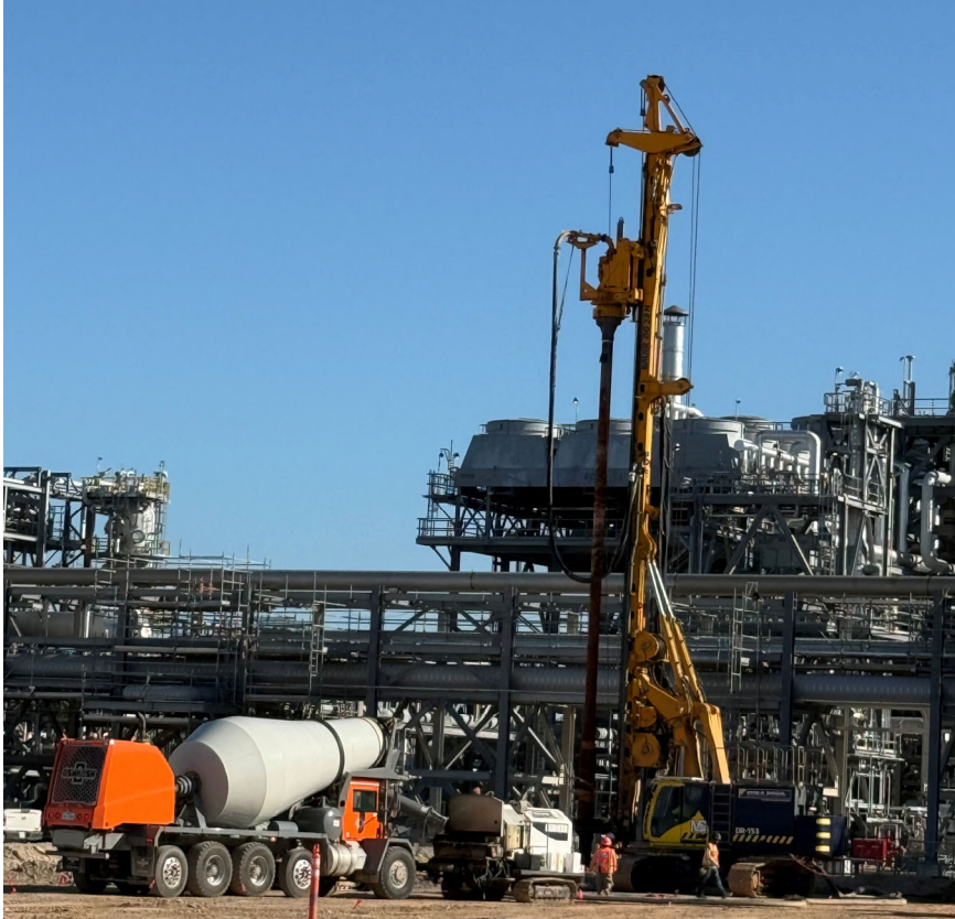
Photo 5: EFG Pile Installation
