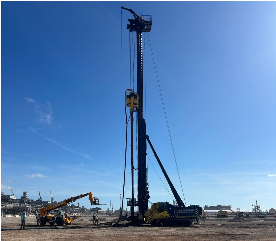
Photo 4: Train 9 Pile Installation
