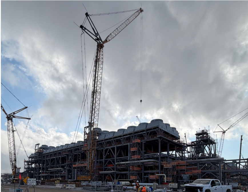
Photo 2: Train 7 Aboveground Piping Installation
