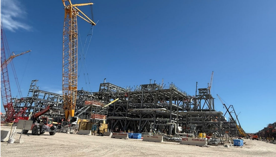
Photo 3: Train 7 Structural Steel
