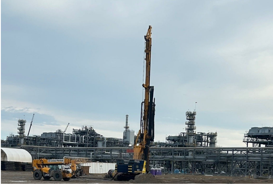
Photo 5: EFG Pile Installation
