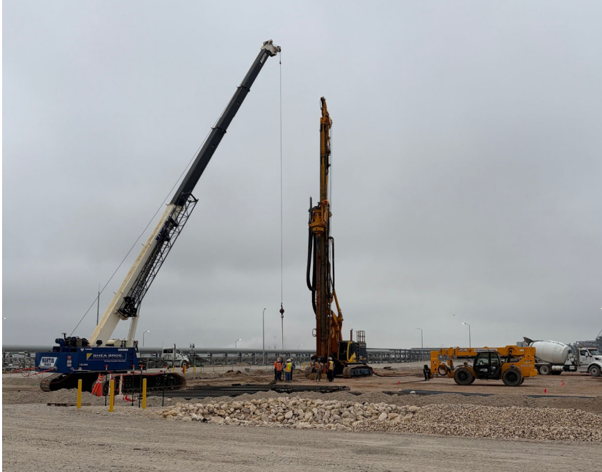
Photo 5: OSBL Refrigerant Storage Pile Installation
