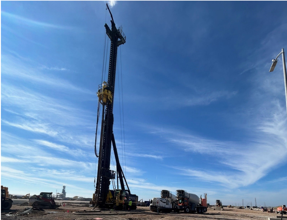
Photo 4: Train 9 Pile Installation
