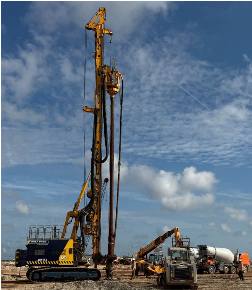
Photo 5: Train 8 Pile Installation
