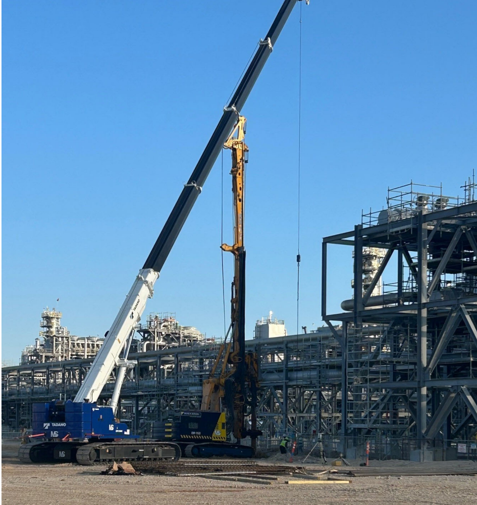
Photo 5: EFG Pile Installation
