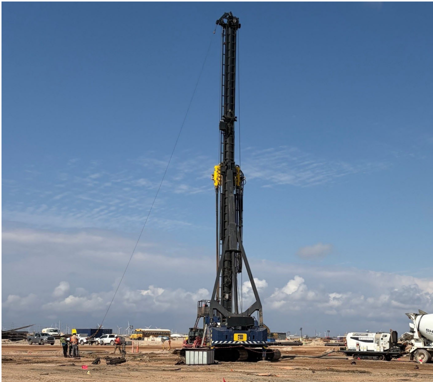
Photo 4: Train 9 Pile Installation
