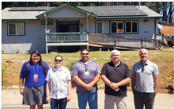
The Karuk Tribe cuts its facilities' energy use by 92% through solar and battery storage. Source: U.S Department of Energy
