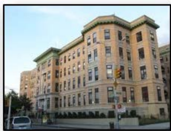
Multifamily Energy Efficiency
