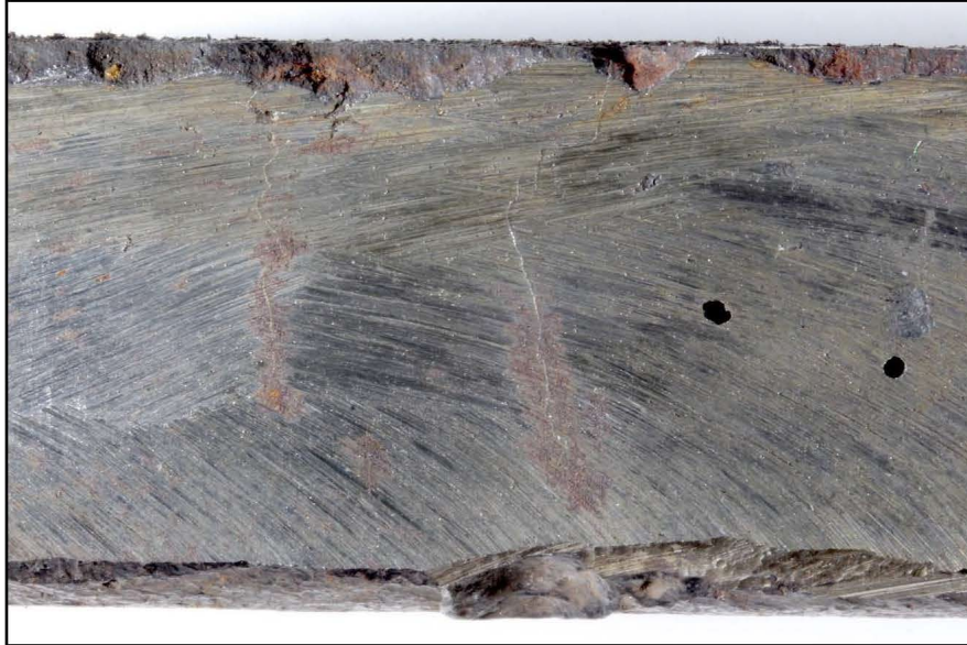
Figure 5. Close-up image of several of the cracks at Region B. A cross-section specimen was prepared through the center of these irregular cracks. Several gas pores are also apparent in this image.
