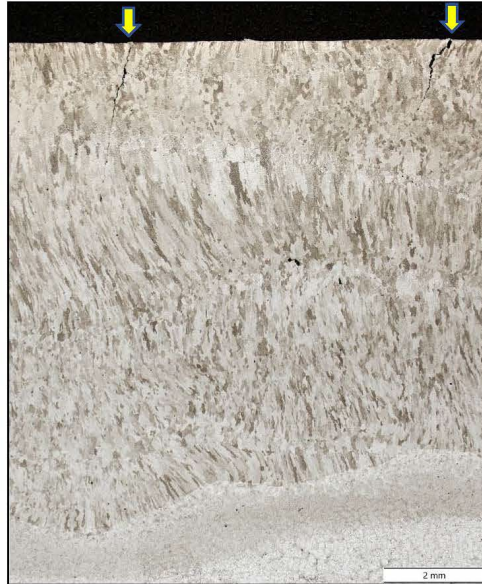
Figure 9. Photomontage of the crack region in Figure 8 after metallographic etching. The cracks were entirely within the weld (arrows). (2% Nital etch, 8.8X)
