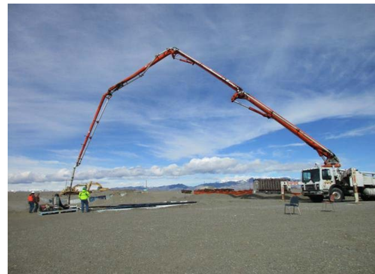
Grouting void spaces in and around cargo containers
