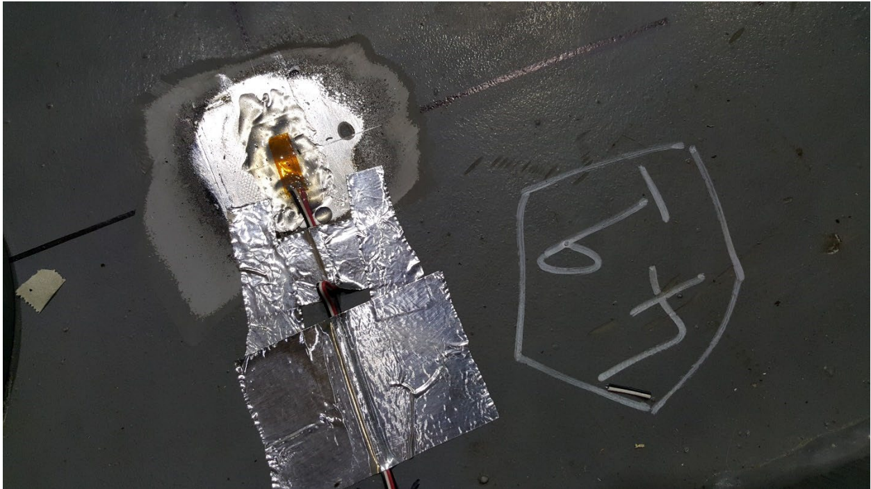
Figure C53. SGDP49 Top of Deck Plate, Longitudinally Centered over B-end Body Bolster, above LH Edge of Center Sill
