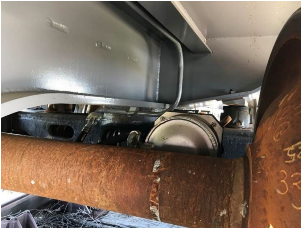
Figure 37. Clearance between Brake Cylinder and Center Sill with Buffer Railcar in 150-foot Radius Curve
