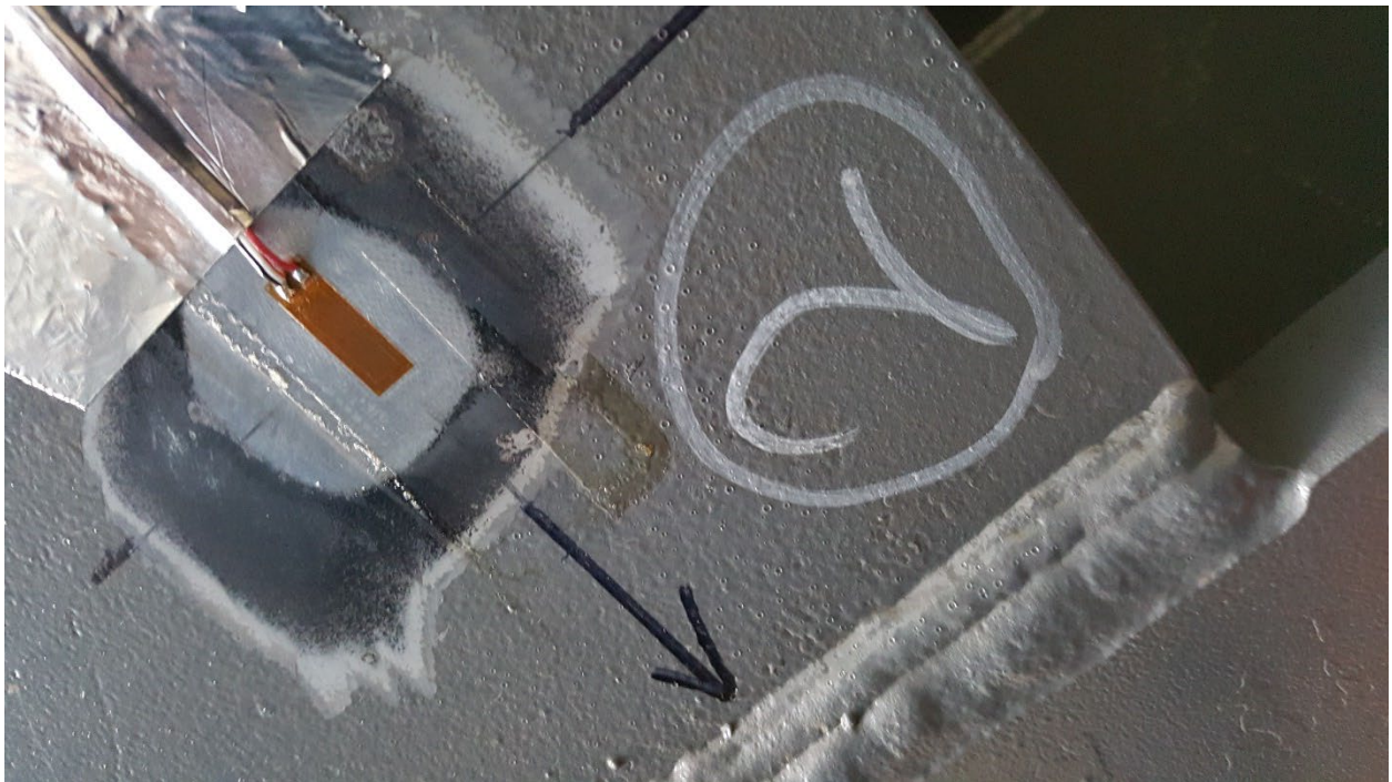
Figure C6. SGBF2 Rear of Bottom Flange of A-end Body Bolster near Center Sill, LH Side
