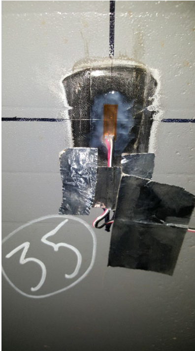
Figure C39. SGBF35 LH Edge of Bottom Flange of Center Sill, Aft of Cross Bearer 1
