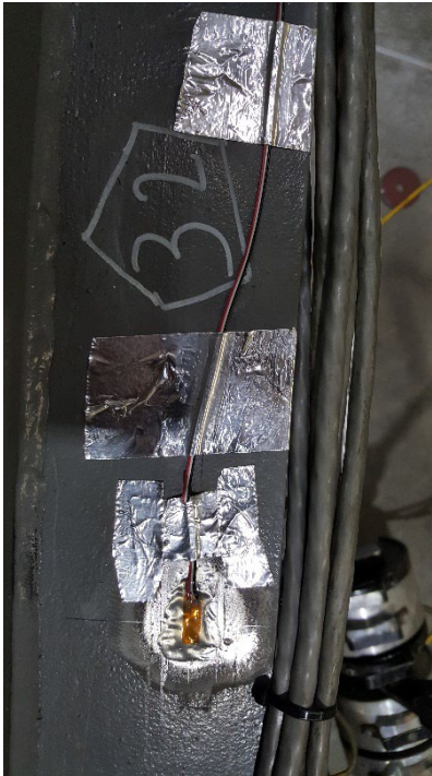
Figure C36. SGDP32 RH Edge of Deck Plate, Aft of Cross Bearer 2
