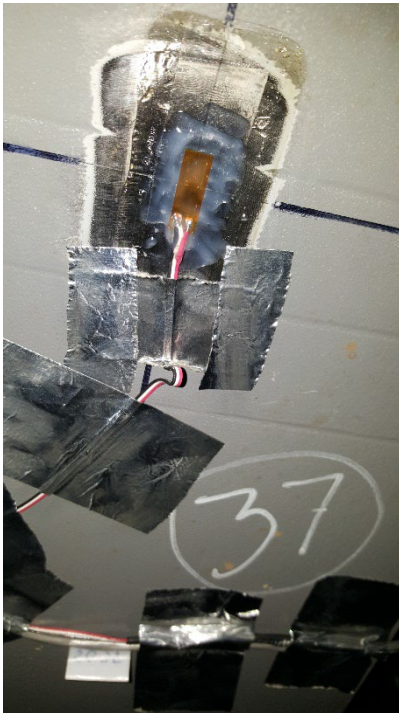
Figure C41. SGBF37 RH Edge of Bottom Flange of Center Sill, Aft of Cross Bearer 1
