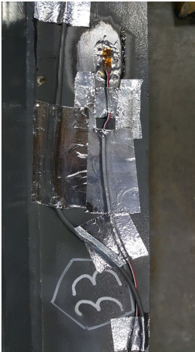
Figure C37. SGDP33 LH Edge of Deck Plate, Forward of Cross Bearer 2
