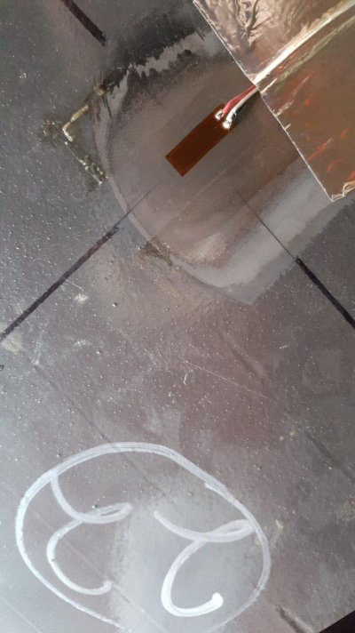
Figure C26. SGBF22 RH Edge of Bottom Flange of Center Sill, Forward of Cross Bearer 6
