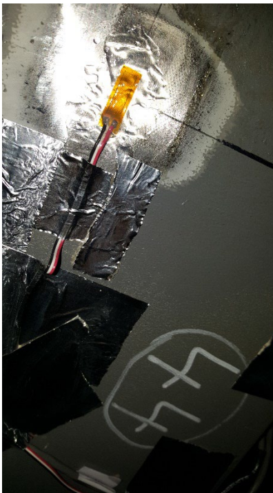
Figure C48. SGBF44 RH Edge of Bottom Flange of Center Sill, Forward of B-end Body Bolster
