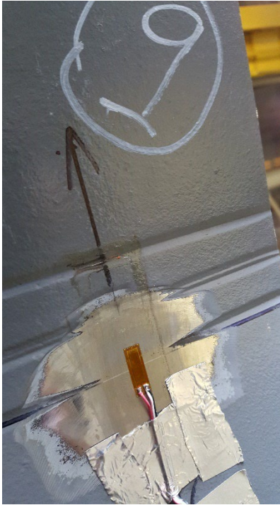
Figure C13. SGBF9 Center of Bottom Flange of LH Side Sill, forward of Cross Bearer Location 7
