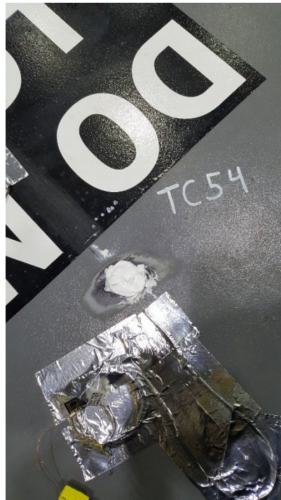
Figure C58. TC54 Bottom Flange of Cross Bearer 4 at Lateral and Longitudinal Center of Car
