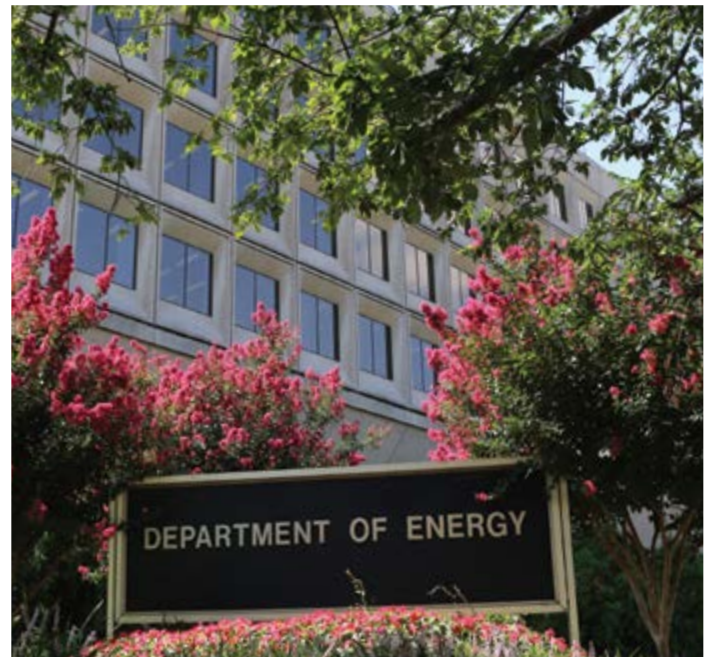
James V. Forrestal Building, Washington, D.C.
