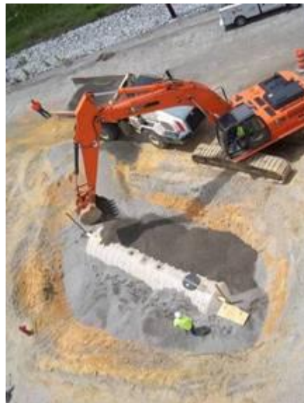
Underground rainwater collection tank for irrigation
