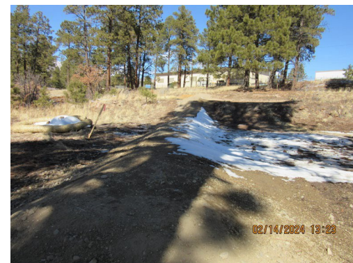
Base course berm (2024)
