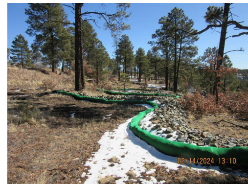
Compost logs (2024) and rock check dams (2015)
