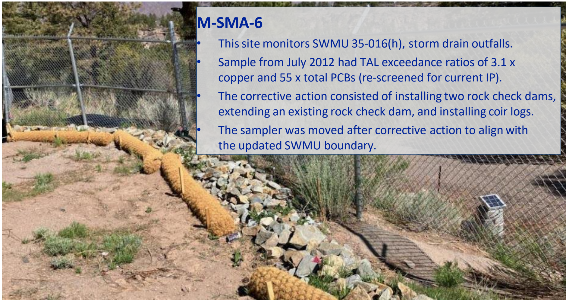
Coir logs M00803140051 and M00803140052, rock berm M00803140031, and sampler at M-SMA-6.
