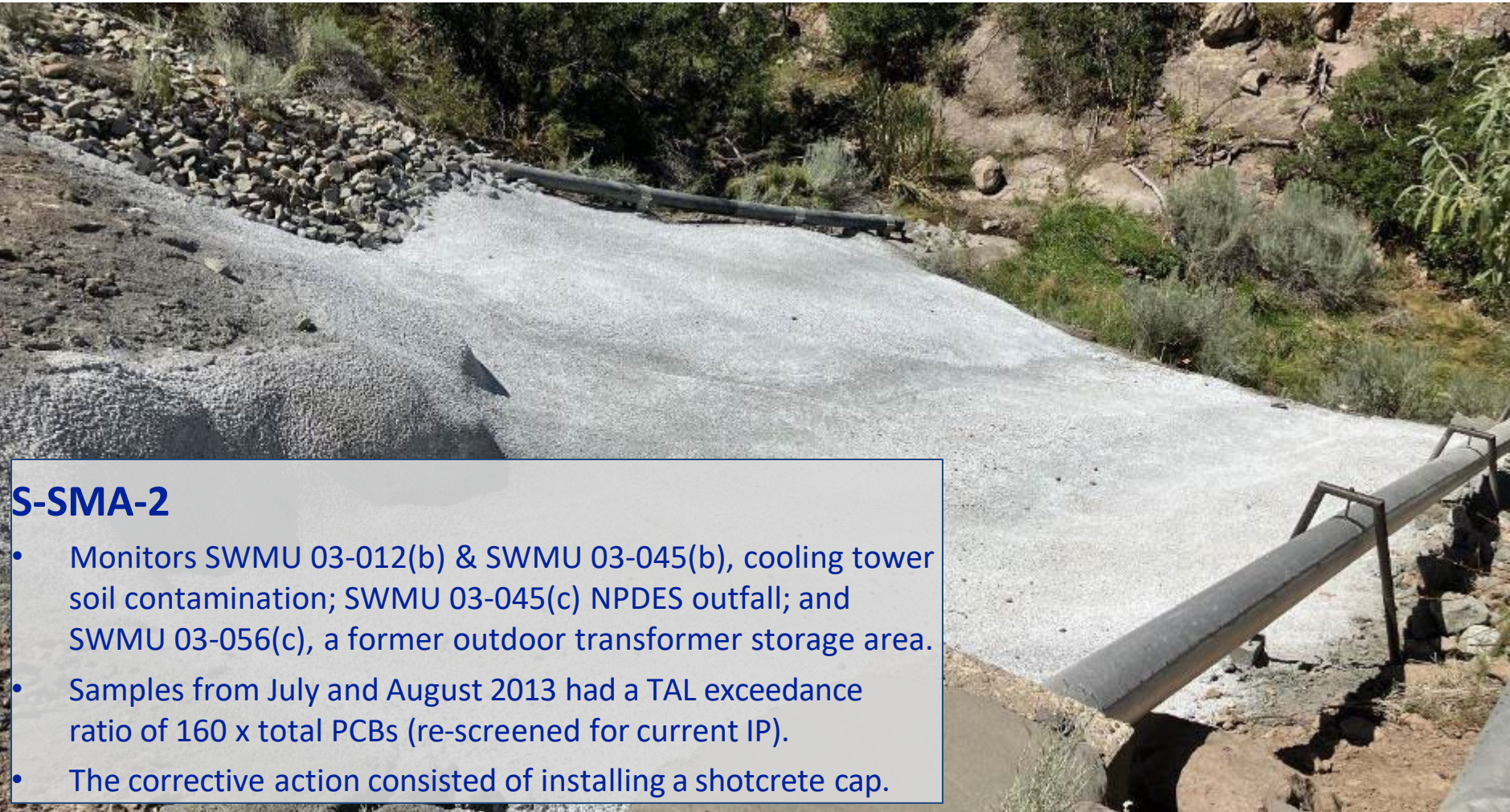
Shotcrete cap S00308060028 at S-SMA-2.
