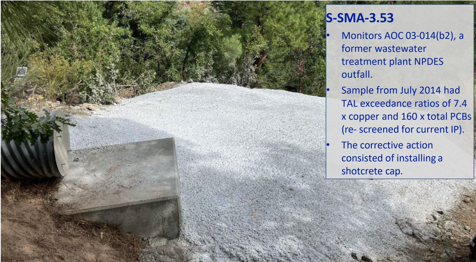
Shotcrete cap S005B08030008 at S-SMA-3.53.
