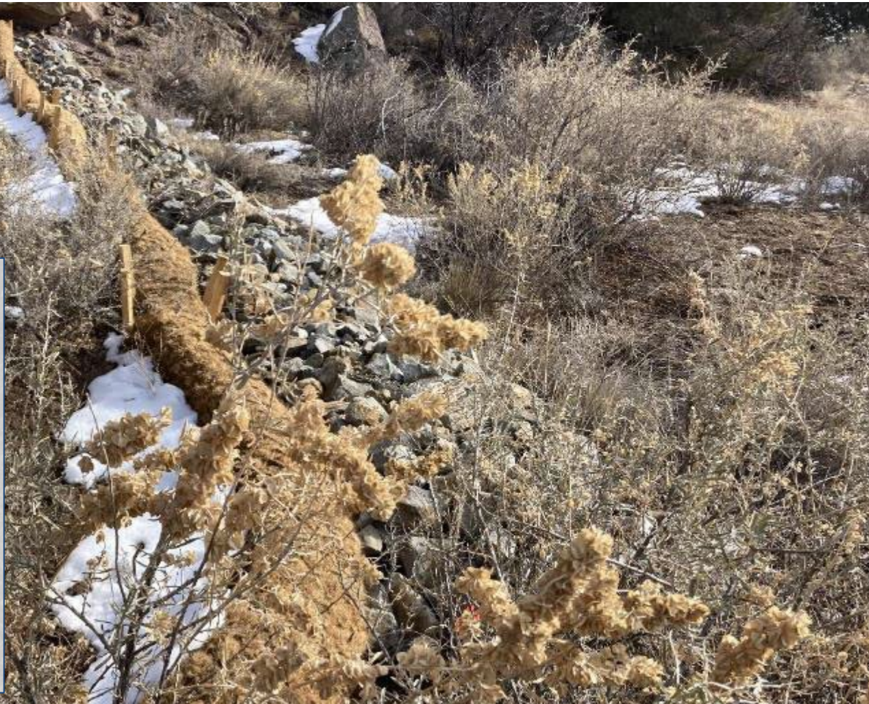
Coir log S01403140024 and rock berm S01403140017 at S-SMA-5.02.
