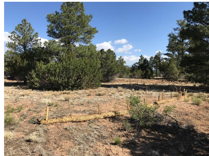
New stormwater controls at W-SMA-11.7
