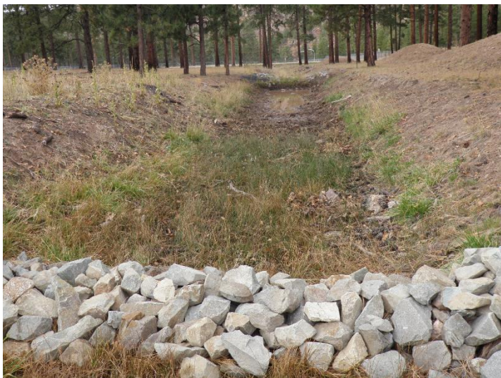
Sediment basin at W-SMA-1.5
