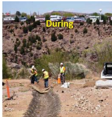
Installation of storm water controls at P-SMA-2.2
