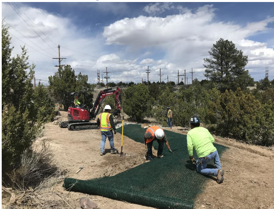
Earthen berm construction at CHQ-SMA-1.02
