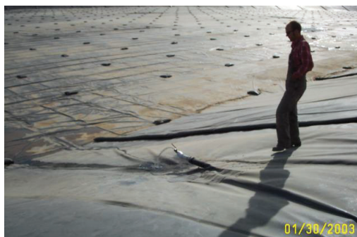
First discharges to pond, 2003
