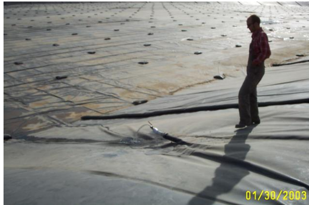
First discharges to pond, 2003
