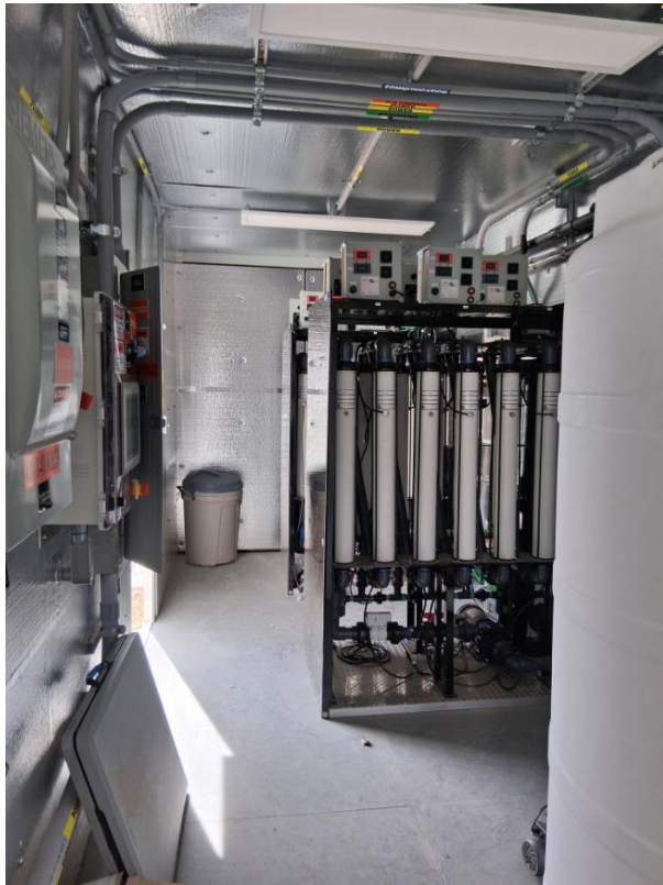
Electrocoagulation system interior
